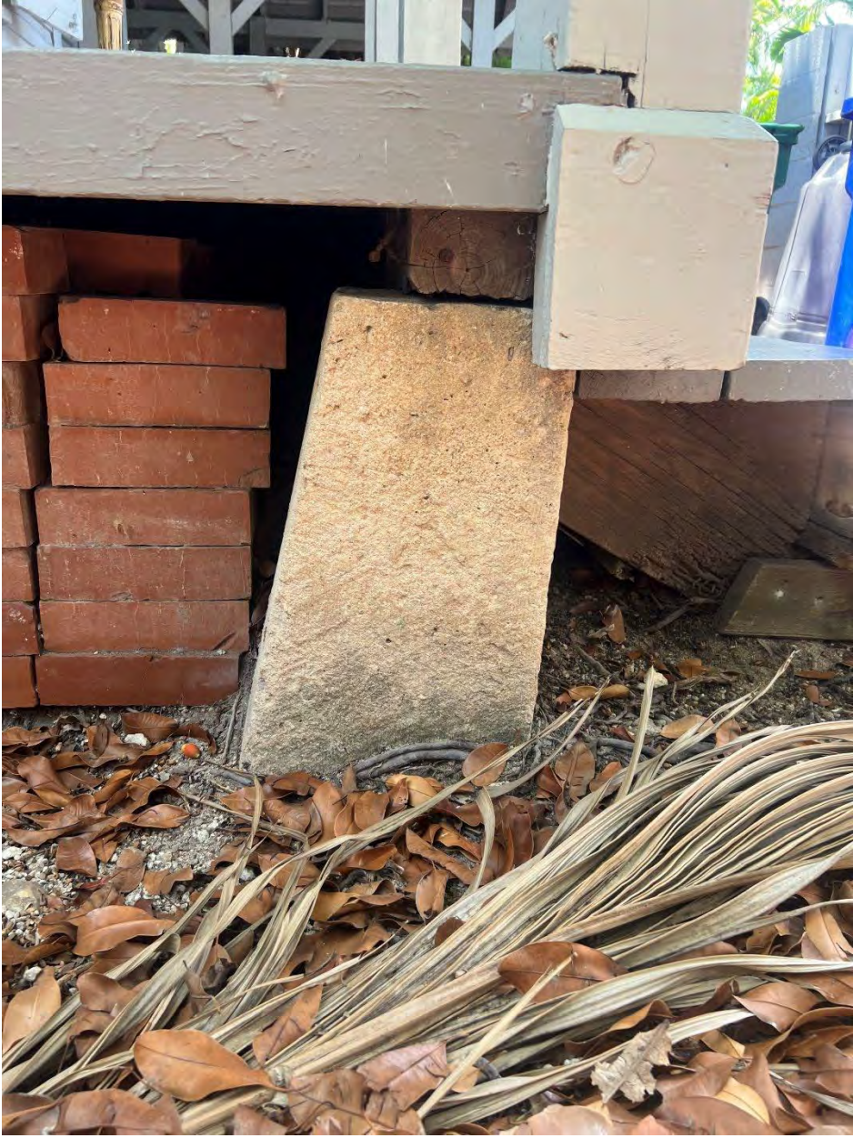
FRONT PORCH FOUNDATION
