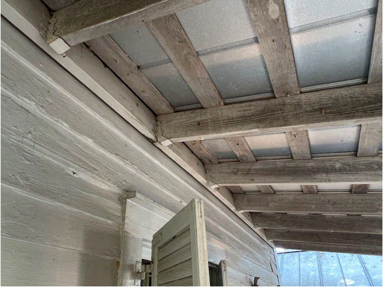
FRONT PORCH ROOF (ALTERED)
