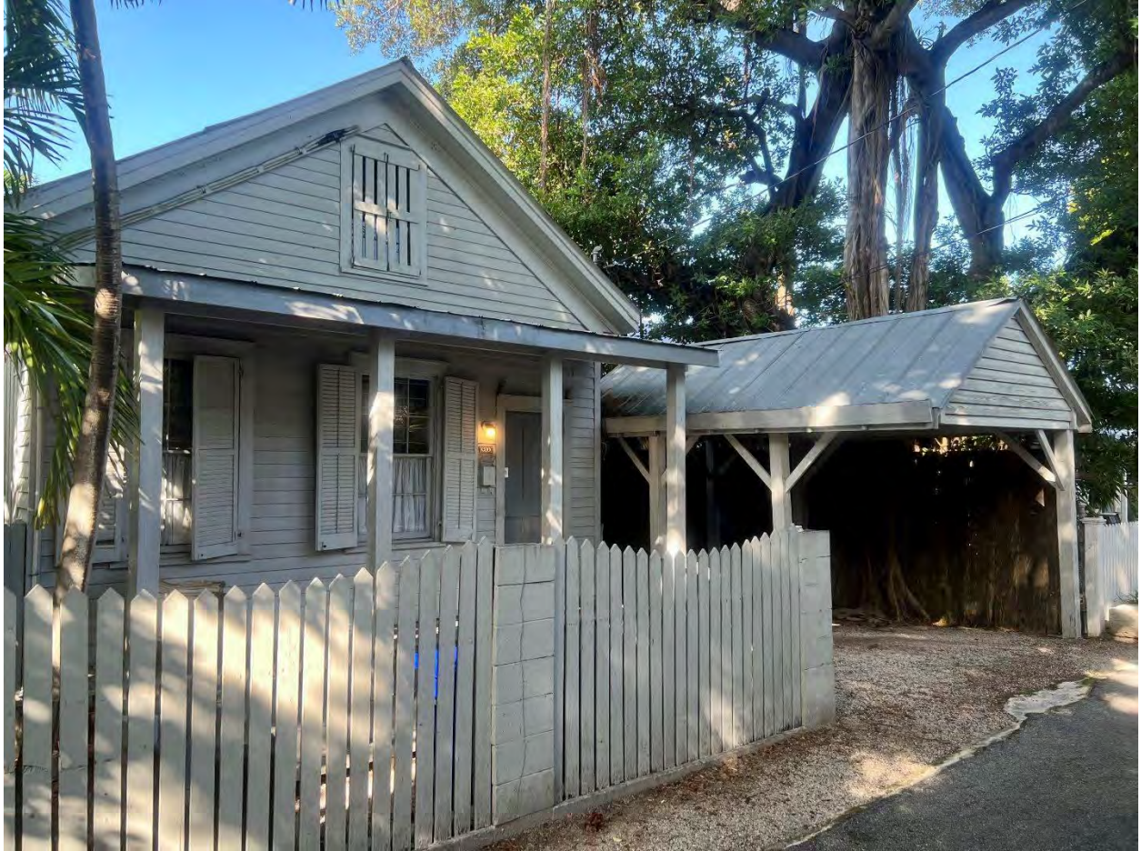
VIEW FROM WATSON STREET HISTORIC STRUCTURE AND CARPORT
