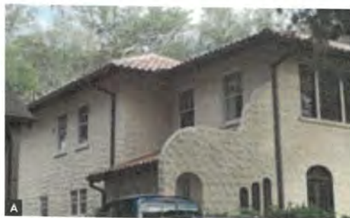
Replacement windows on side of residence.
