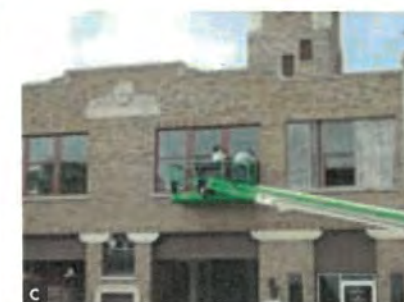
A) North-Window; B) West Wall After New Window; C) Window Installation on Facade
