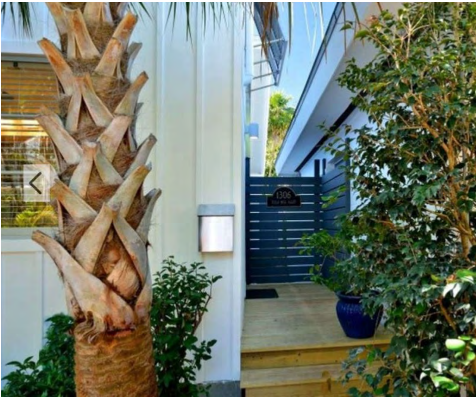
1306 Villa Mill – front entry showing encroachment by 638 United St.
