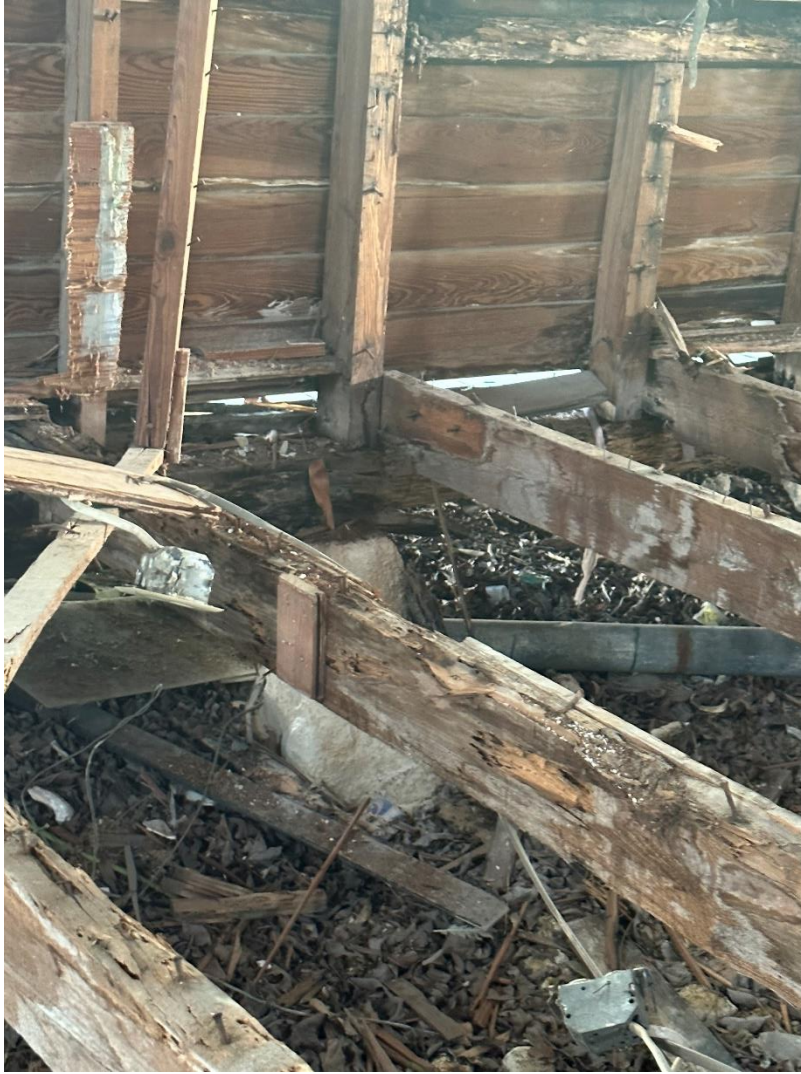
Photograph 4: Photograph of the interior joists, rim beam and window framing.
