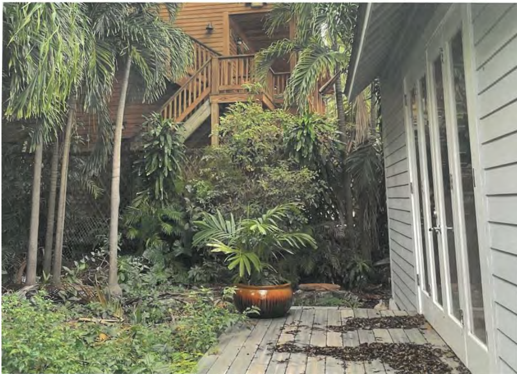
South side and rear elevations.
