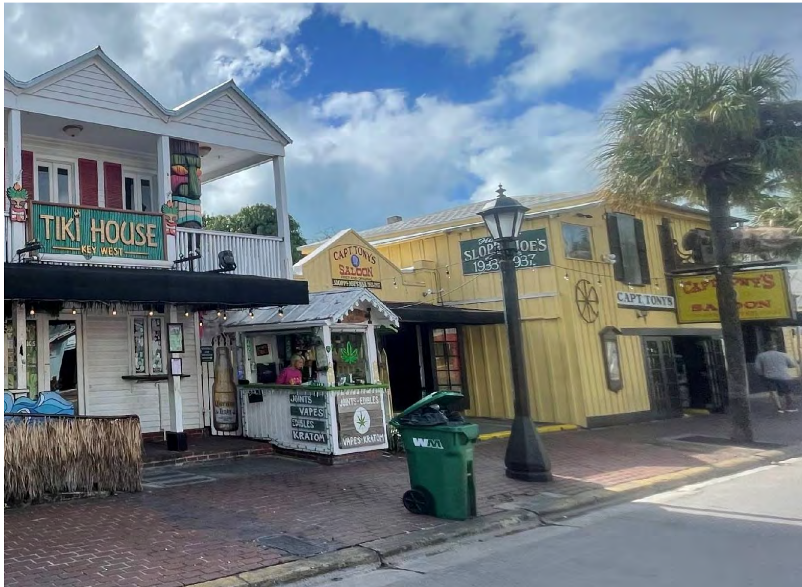
430 GREENE STREET RIGHT NEIGHBORING PROPERTY SIDE VIEW
