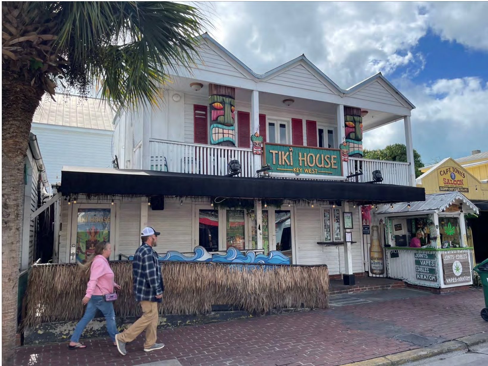
430 GREENE STREET FRONT VIEW
