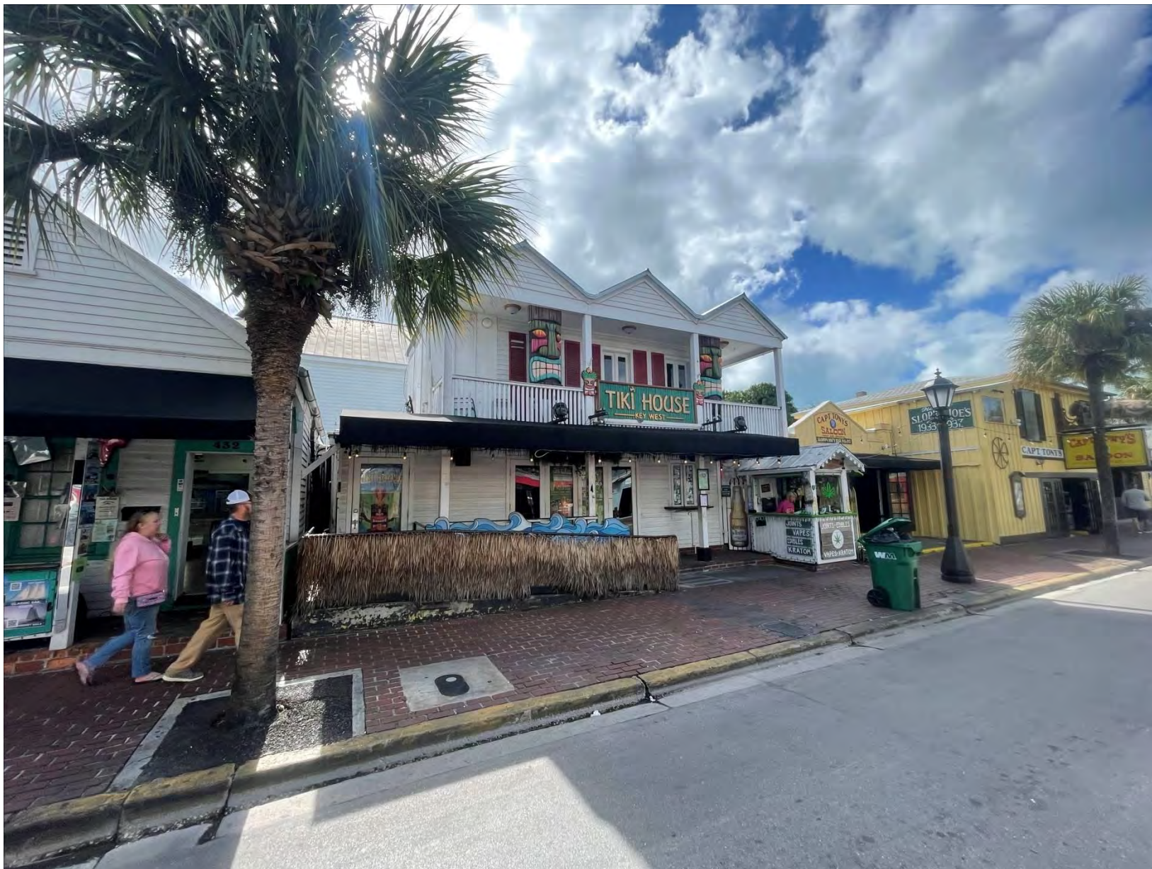
430 GREENE STREET FRONT VIEW
