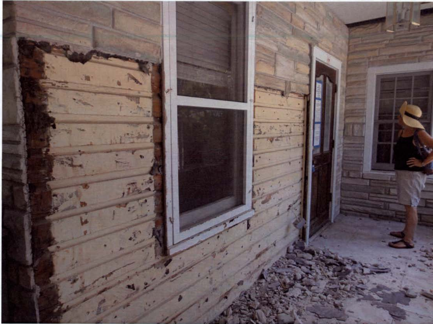
(photograph showing historic novelty siding below existing cementitious exterior finish)
