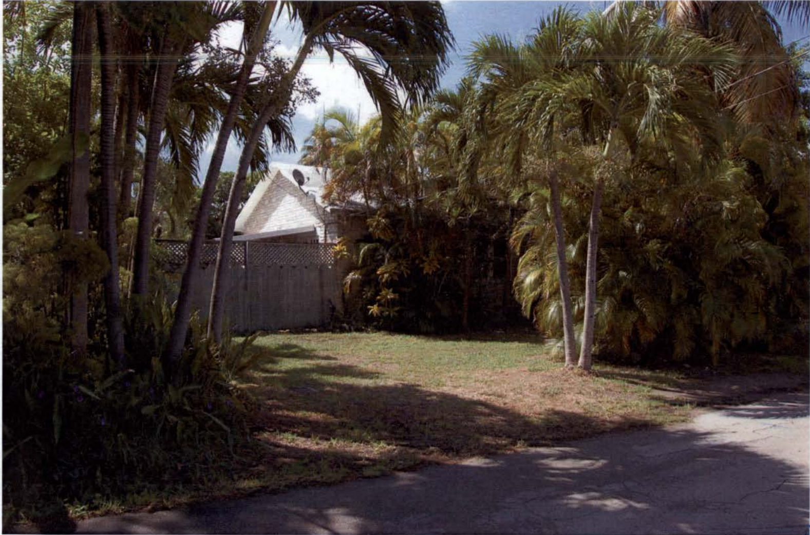
View of property from Washington Street looking South West
