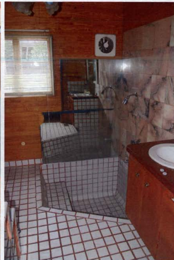
Sunken tub in non historic addition. Finished floor in this addition is 5" below historic structure.
