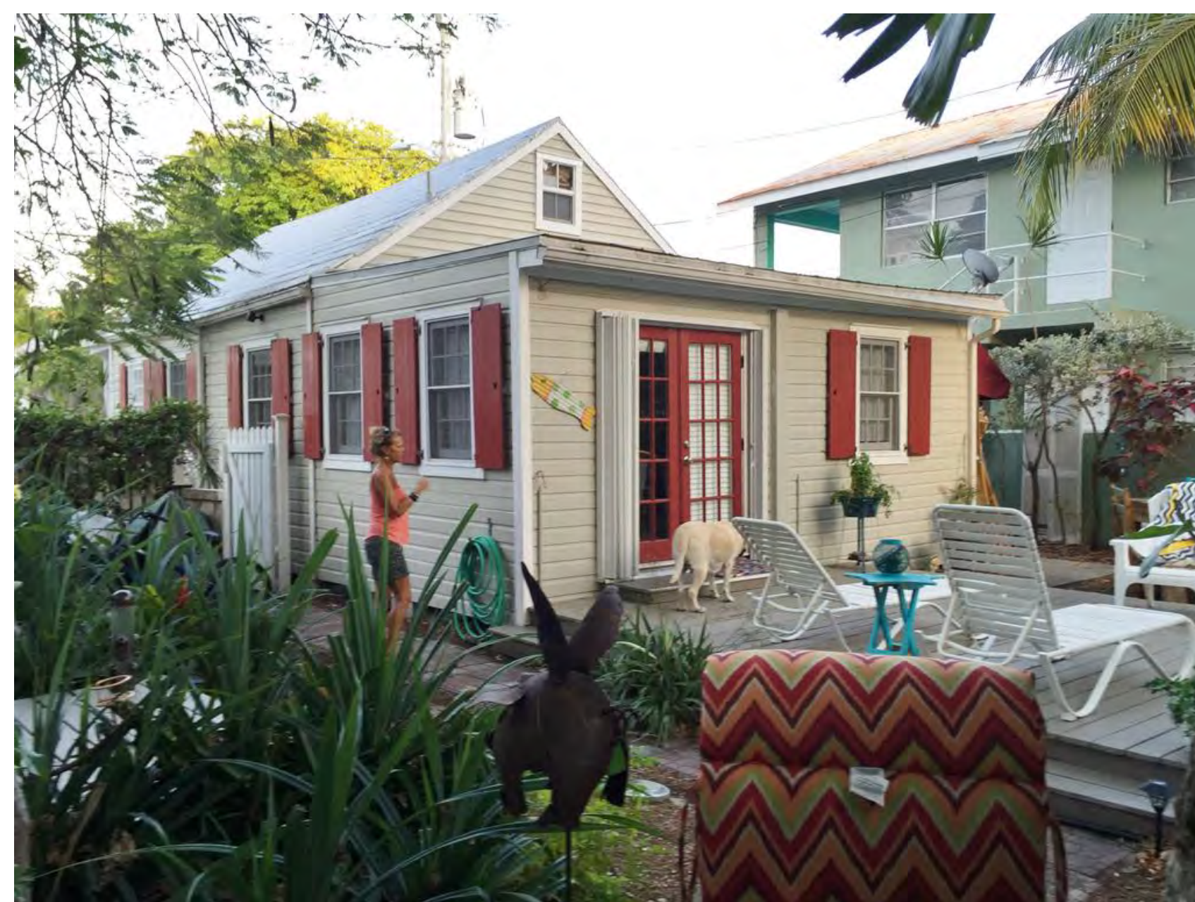
BACK ELEVATION, PHOTO 3
