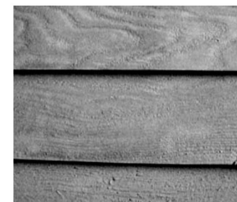
CONCRETE FORMLINER WALL FINISH NTS
