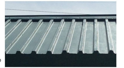
CONCRETE FORMLINER ROOF FINISH NTS
