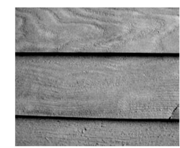
CONCRETE FORMLINER WALL FINISH NTS
