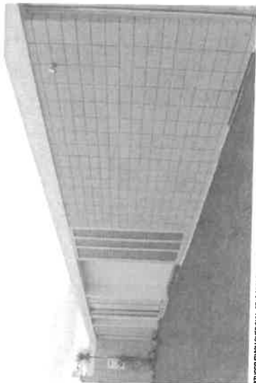
STUCCO FINISH OVER CMU - STACK BOND PATTERN
