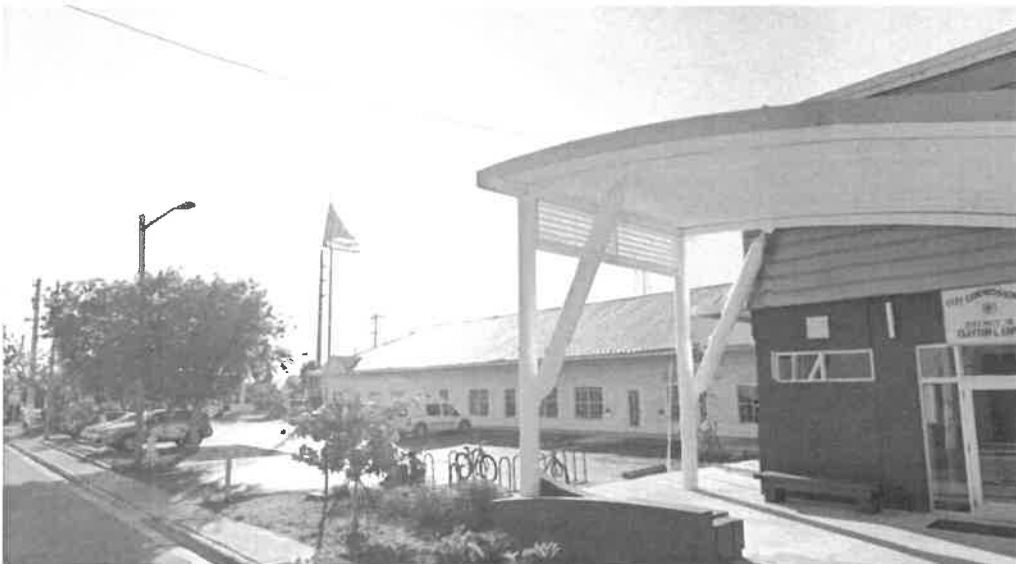
The existing Annex Building.
