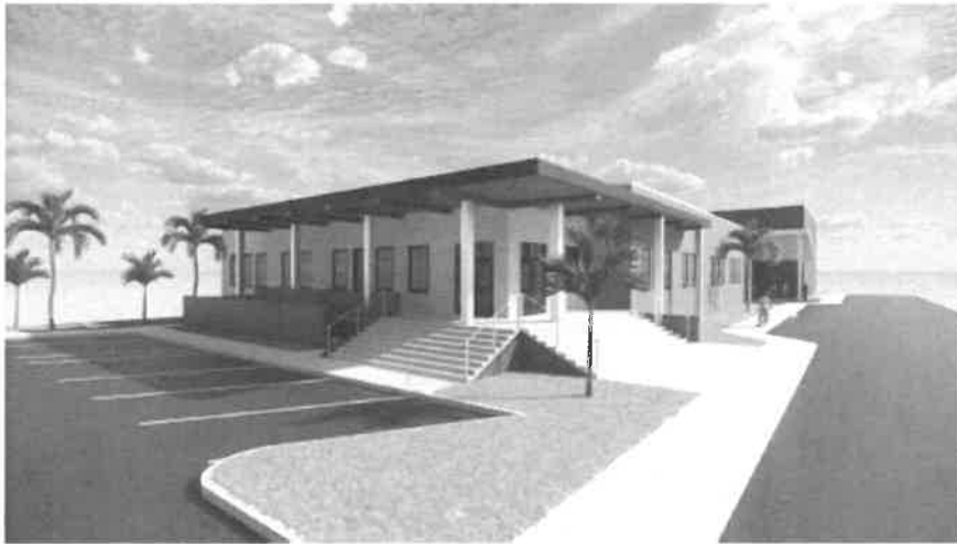
2 FRONT ENTRANCE VIEW
