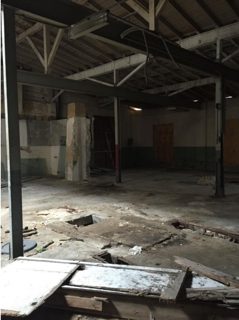
PHOTO 1: Interior of buildings at the Site
