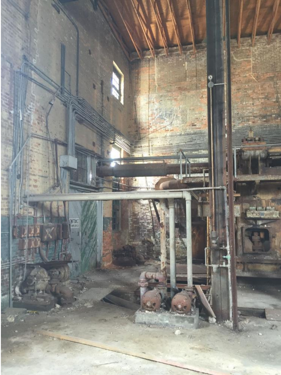
PHOTO 7: Interior of buildings at the Site
