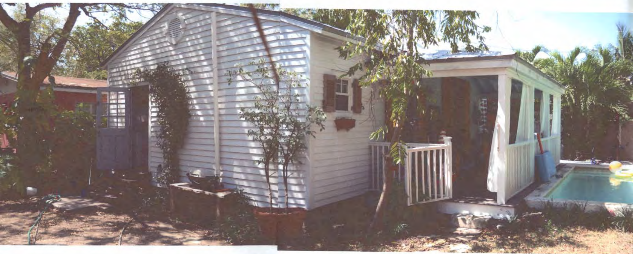
REAR OF EXISTING BUILDING
