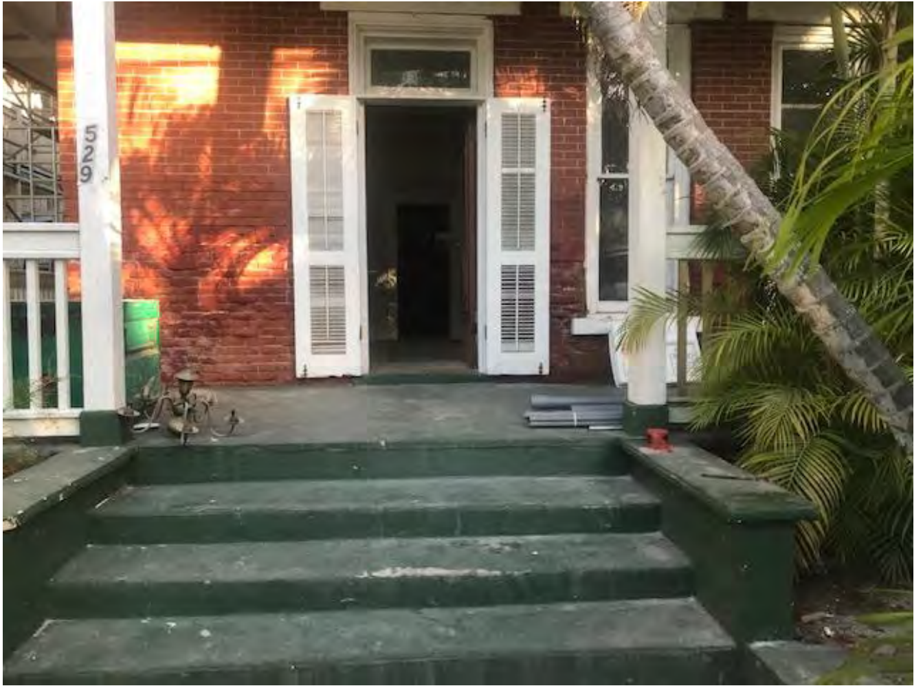
Current conditions, entryway.
