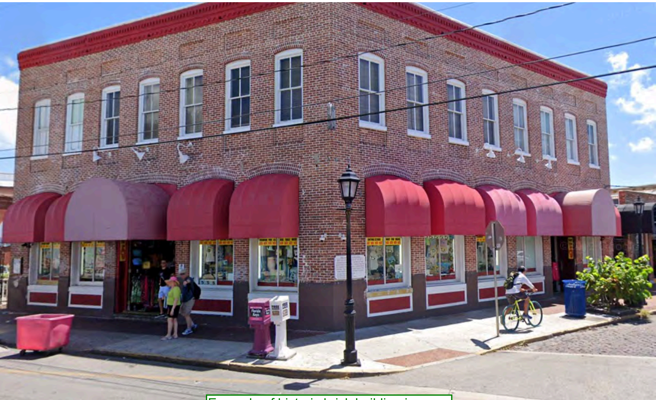
Example of historic brick building in historic Key West with similar stucco repair. 427 Front St.
