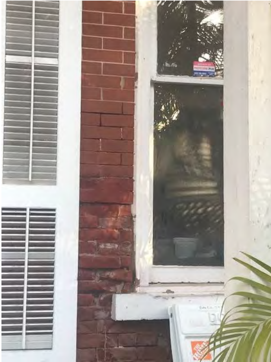
Current conditions, detail front wall.
