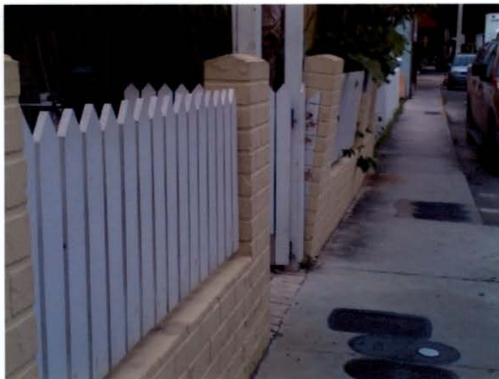
Wall in foreground is unaffected and will not be replaced.
