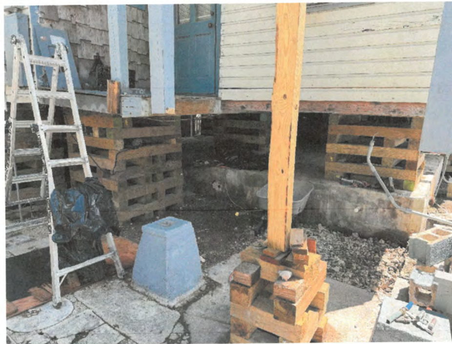
Elevated to new FEMA Flood
