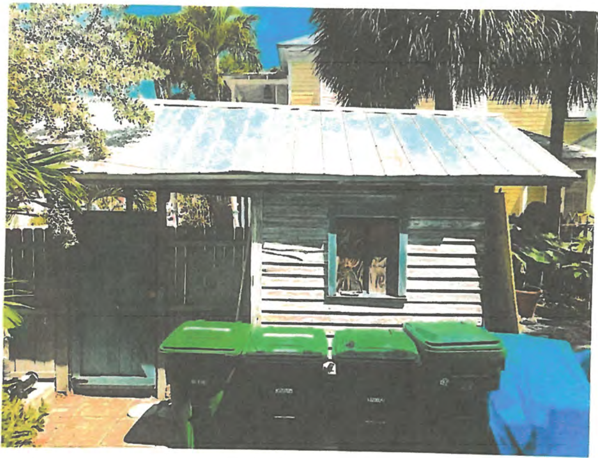
Shed moved from current location and elevated to level of pool deck. Size 13' X 23' vs current size of 11'-3" X 16'-1/2"
