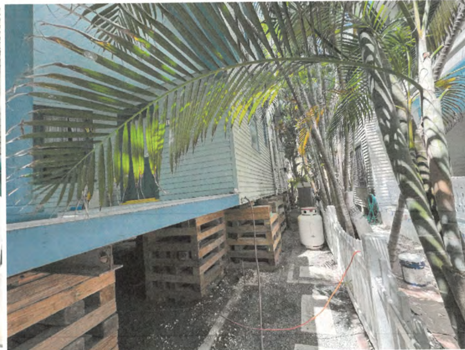
Elevated to New FEMA Flood
