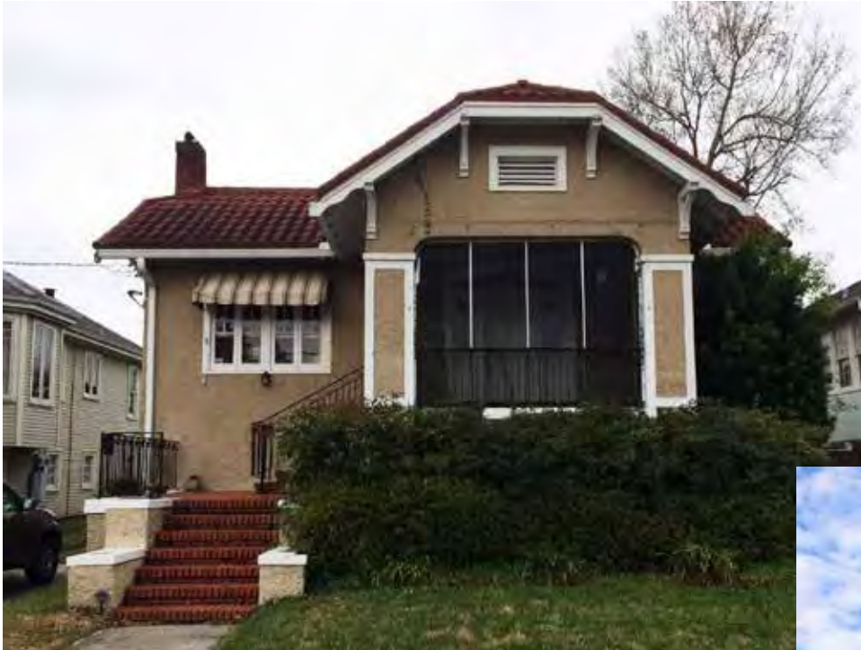
(a) Photo: Rubion Construction Co., LLC
