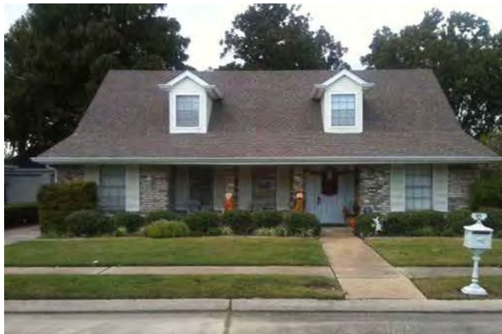
(a) Photo: Rubion Construction Co., LLC
