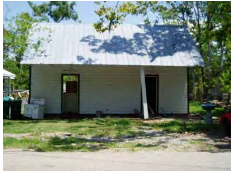
(a) Photo: Rubion Construction Co., LLC
