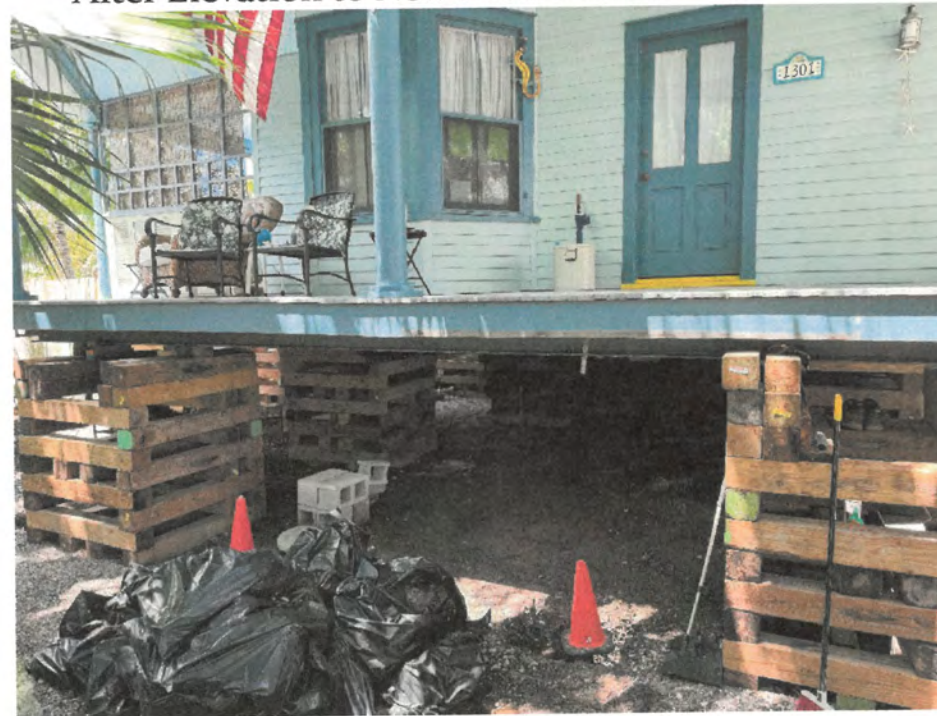
After Elevation to New FEMA Flood
