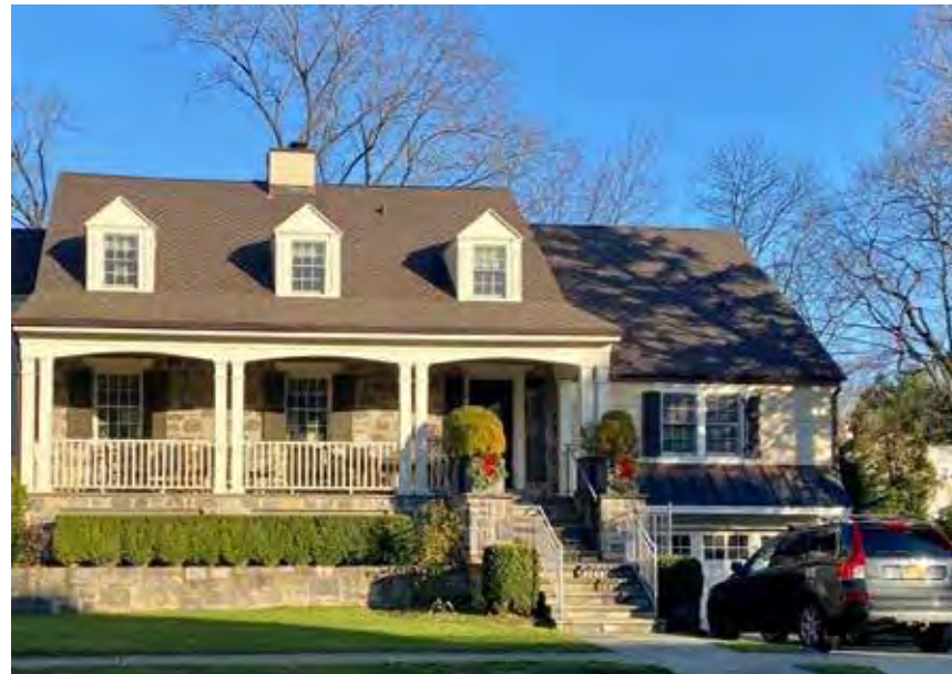
[93] This home has used elevated planting beds across the front of the house to bring the landscaping up higher and help screen the change in height. The stairs are stone, to blend in with the foundation and the planters, and a landing breaks up the long run of stairs at a point that aligns with the top of the planters. This provides a visual reference point for what was the original foundation height. The garage remains at grade level. Photo: FloodSavvy.com
