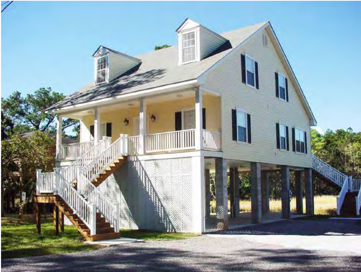
[82] Little can be done to mask or alter the appearance of a tall foundation. Once a building has been elevated the equivalent of a story or more, the overall proportions and scale of the building is often changed, resulting in diminished historic character. Photo: Courtesy of the Southern Forest Products Association
