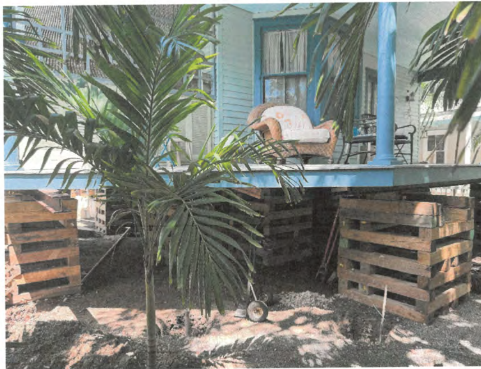
Elevation to New FEMA Flood
