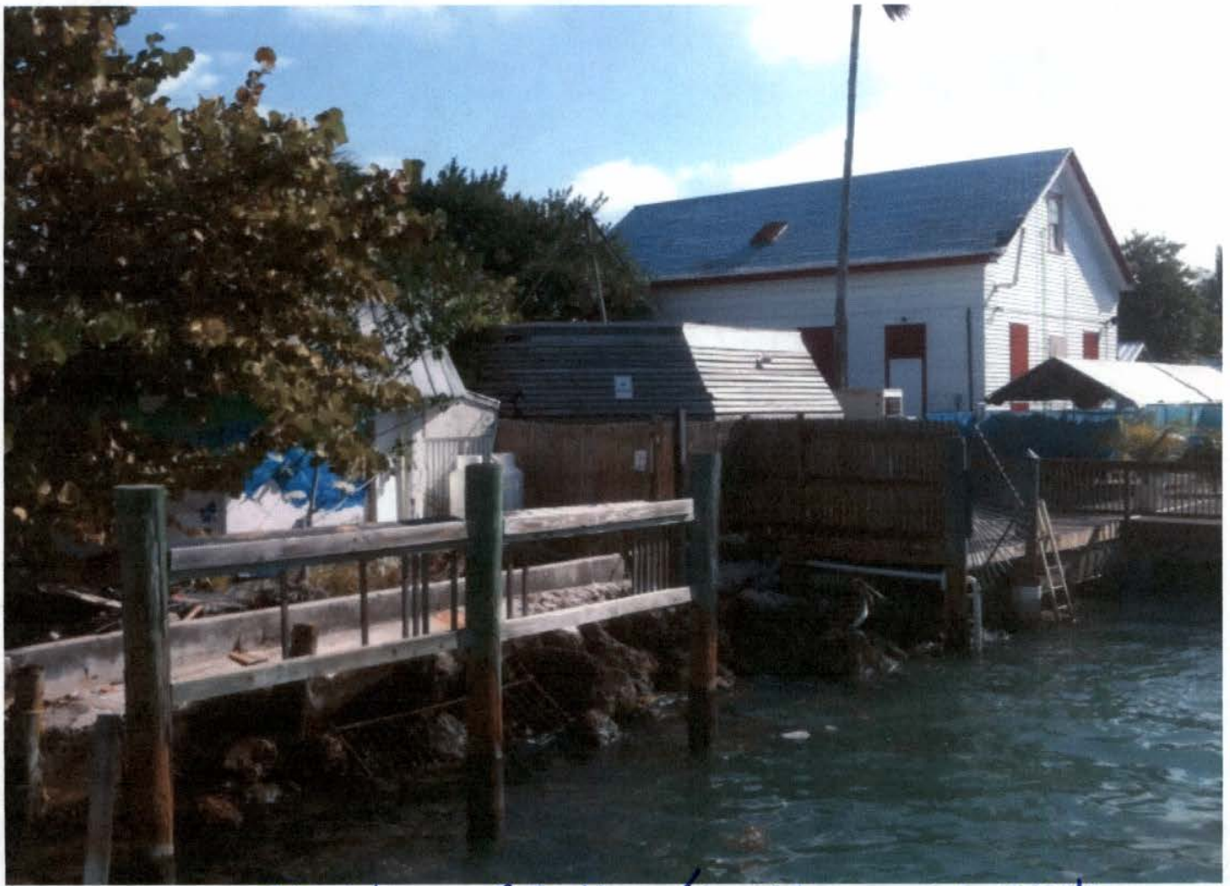
EXISTING BROKEN/ROTTED DECK BEHIND CISTERN
