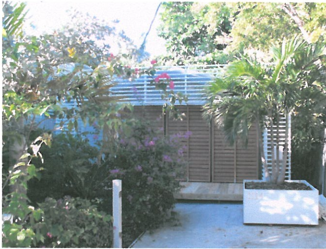
Previous renovation with shutters down.
