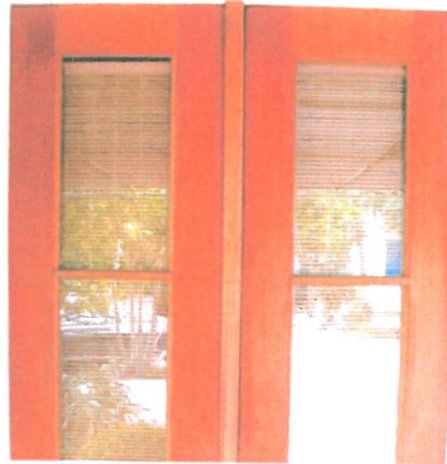
Existing wood doors
