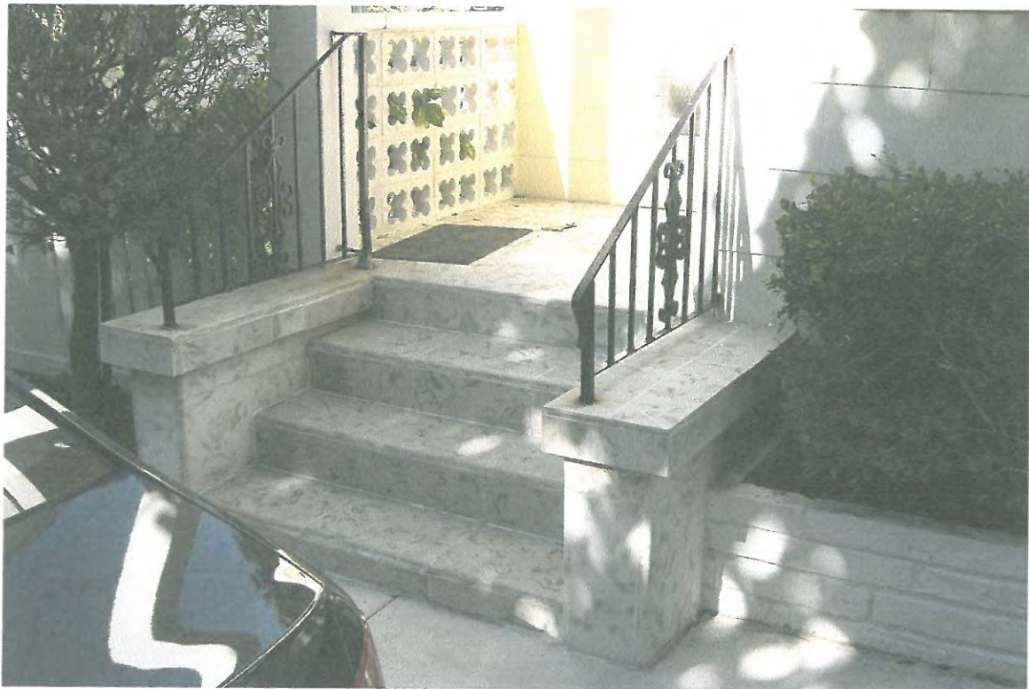
FRONT PORCH STEPS 1117 STUMP LN.
