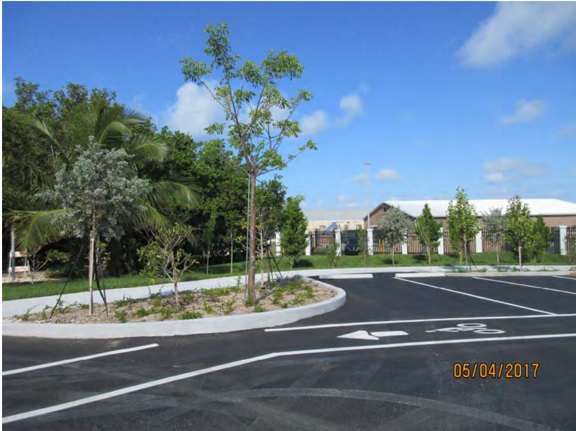
West side of new entrance
