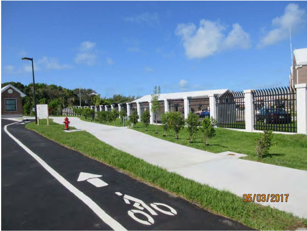
west side of new entrance
