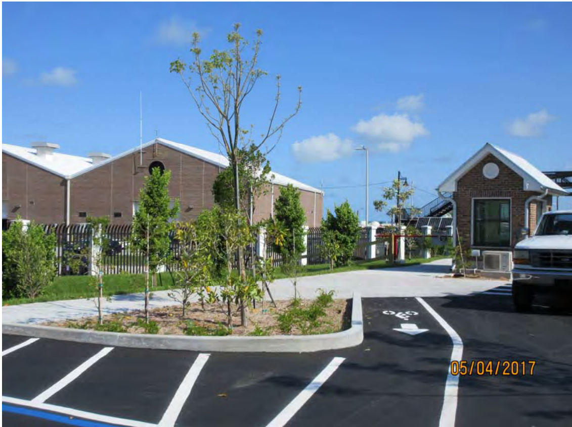
West side of new entrance
