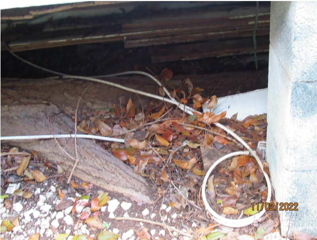
Photo showing tree roots under structure, view 2.
