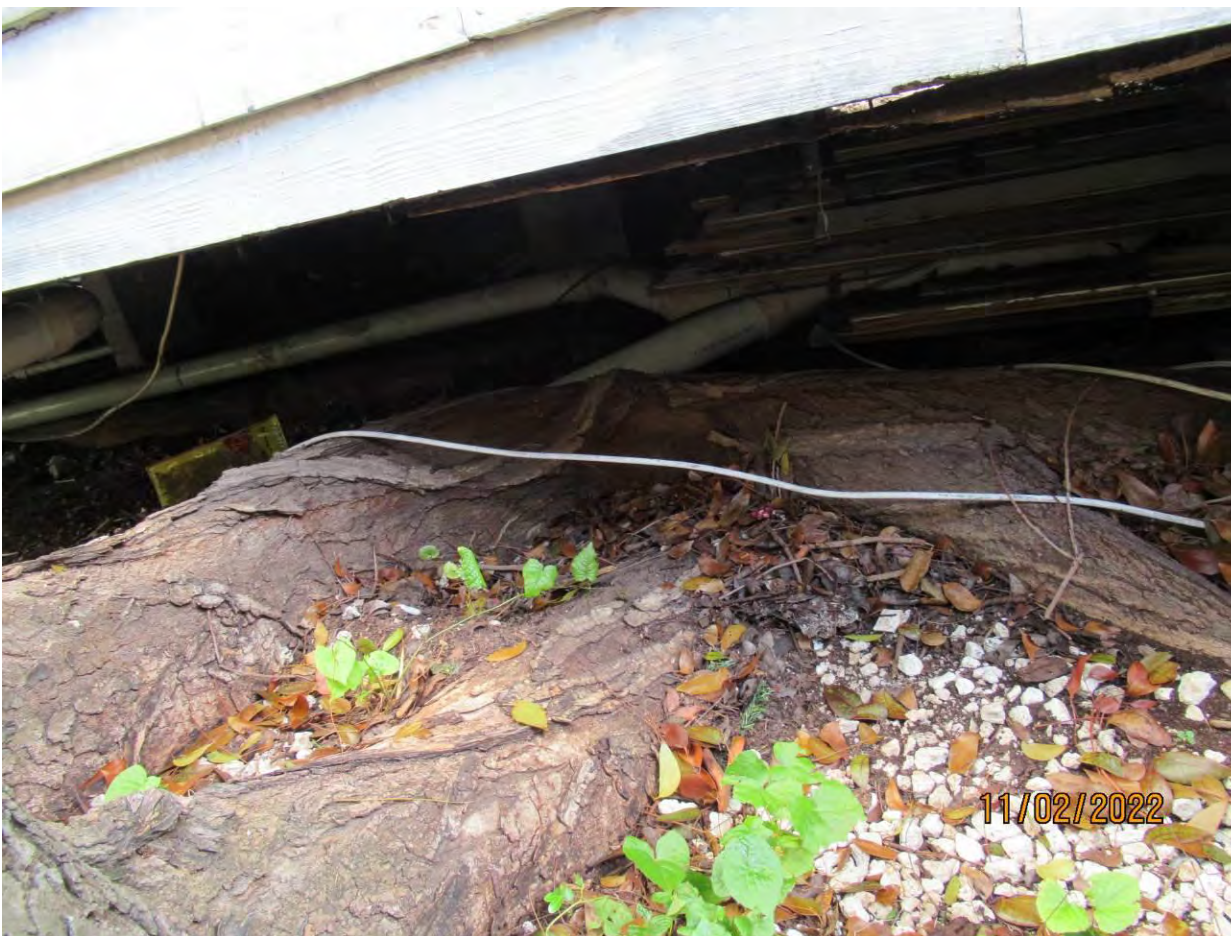
Photo showing tree roots under structure, view 1.
