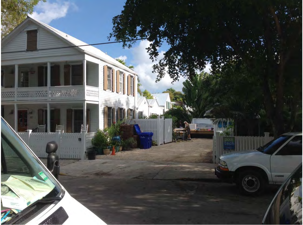
EXISTING CURB CUT, ROLLING GATE AND DRIVEWAY
