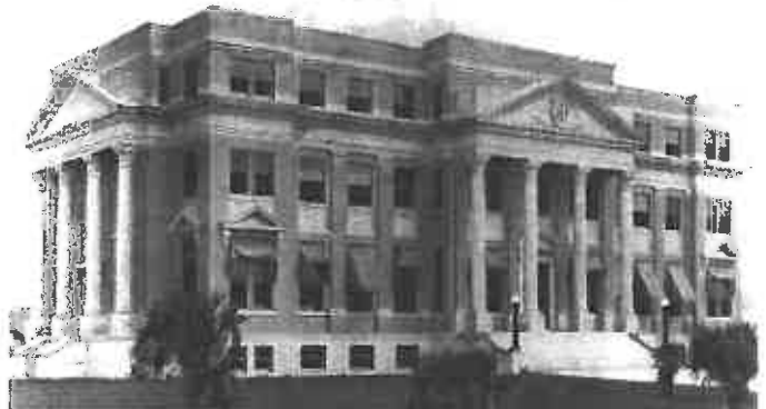
Above: Originally built in 1916, the four-story, 40,000-sq.ft. Palm Beach courthouse was a tour de force of Neoclassical architecture. The architect Wilber Burt Talley designed a granite base, brick and stone façades, soaring Indiana limestone columns and Corinthian capitals that held up triangle pediments, and a dentil molding below the cornice. Photo: historic postcard
