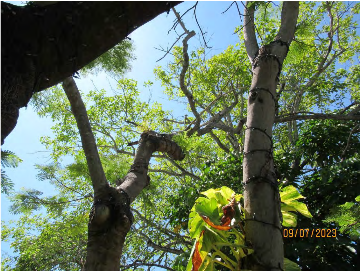
Two close up photos of canopy branches with decay, views 4 & 5.
