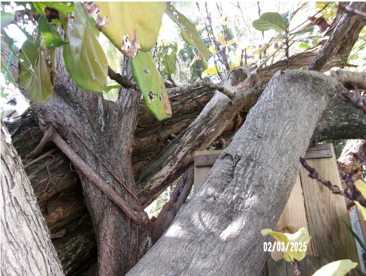
Photo of tree trunks on fence- showing some decay.
