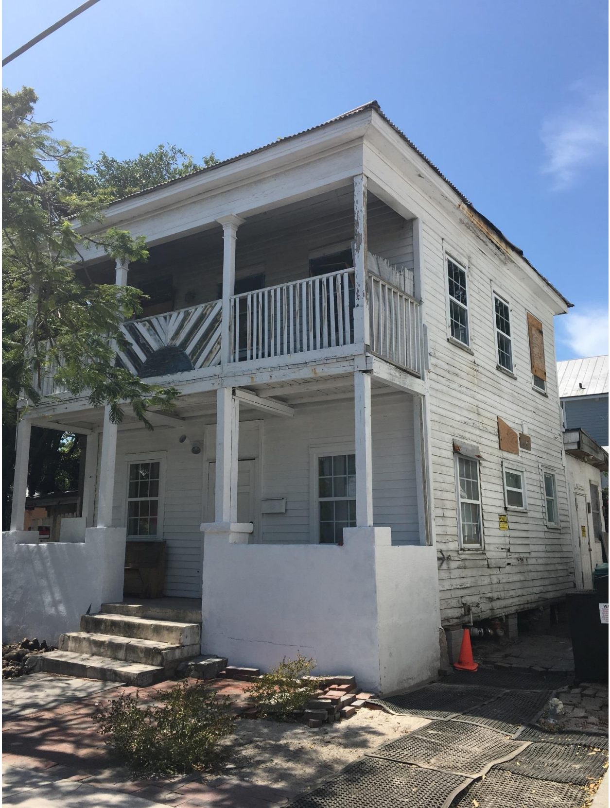
221 Petronia Street, Key West, Florida 33040 SITE VISIT – 3/31/2016
