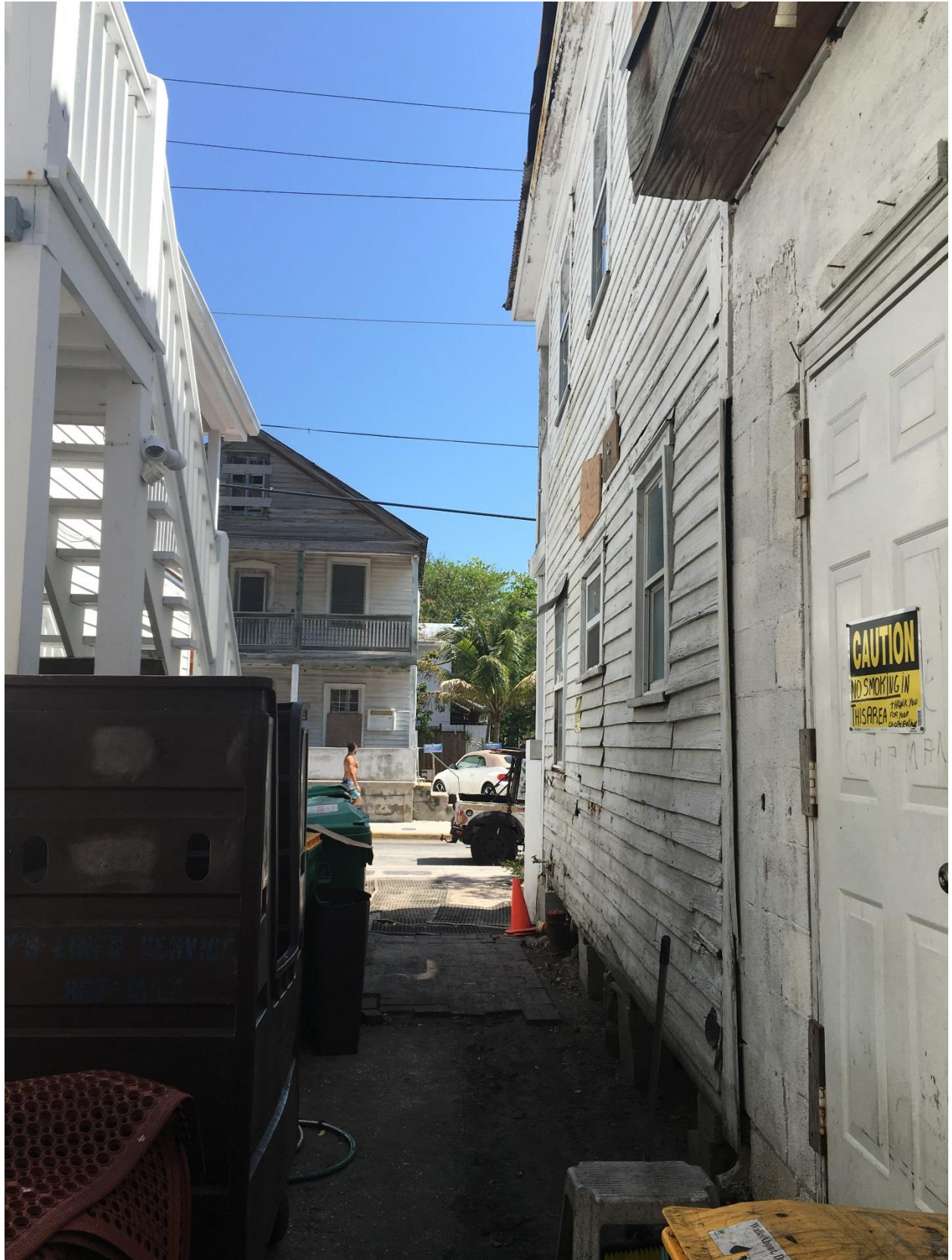
221 Petronia Street, Key West, Florida 33040 SITE VISIT – 3/31/2016
