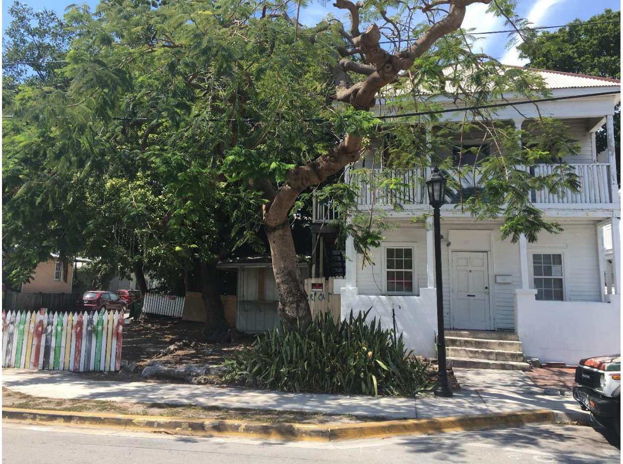
221 Petronia Street, Key West, Florida 33040 SITE VISIT – 3/31/2016
