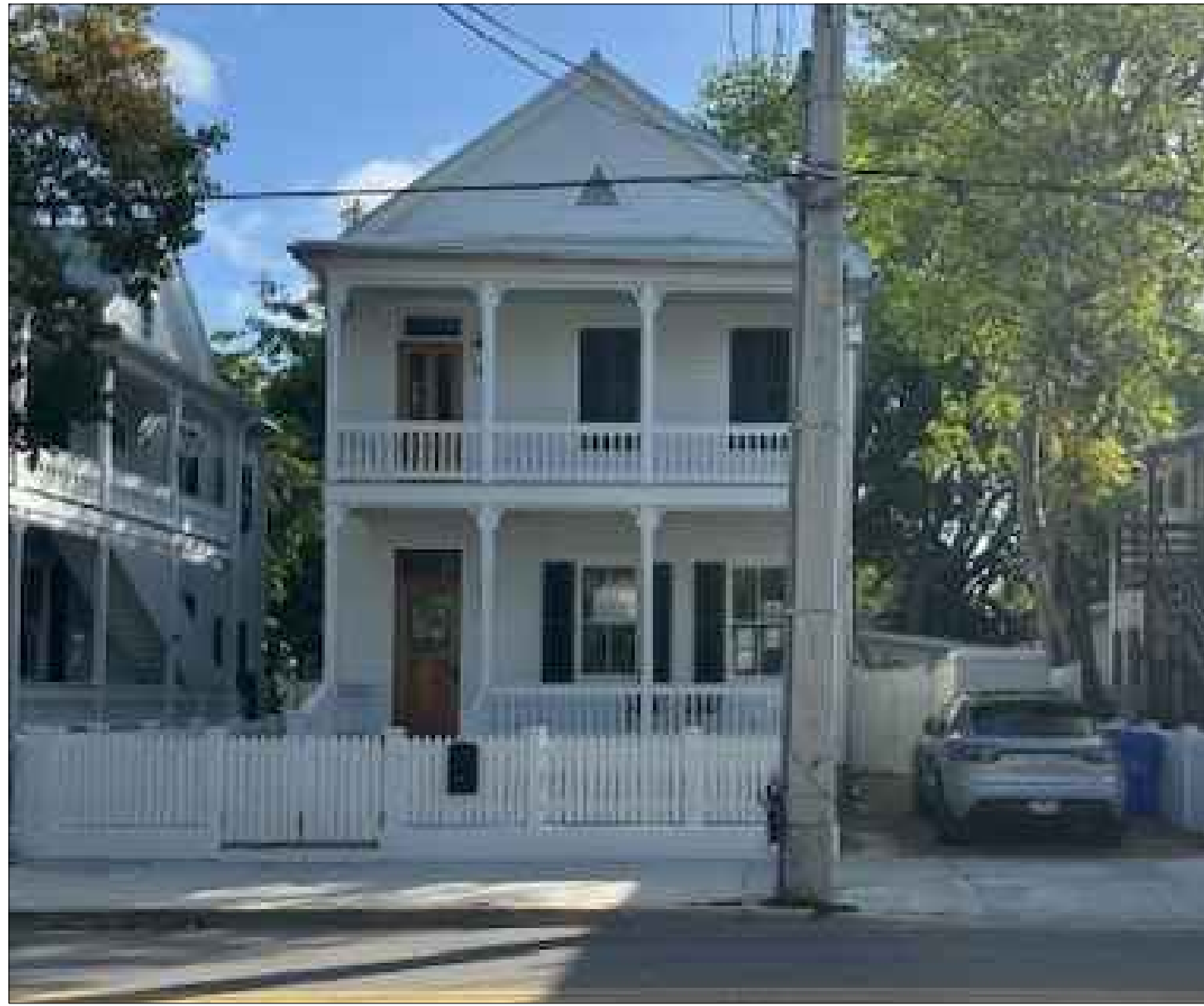
6 VIEW FROM STREET (EXISTING WEST ELEVATION) A7 SCALE: N.T.S.
