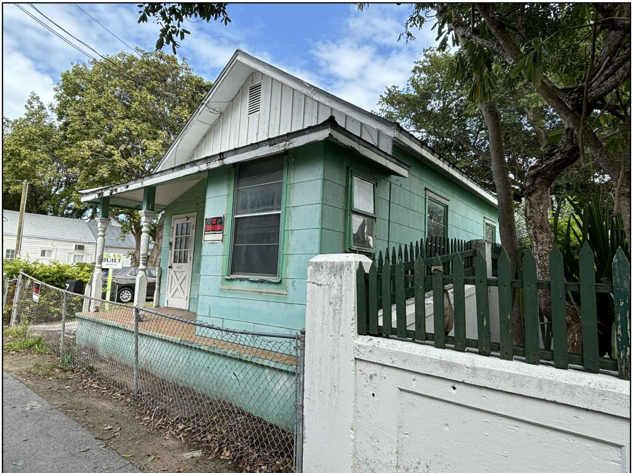
VIEW FROM SIDE OF THE HOUSE (EXISTING SOUTH ELEVATION)
