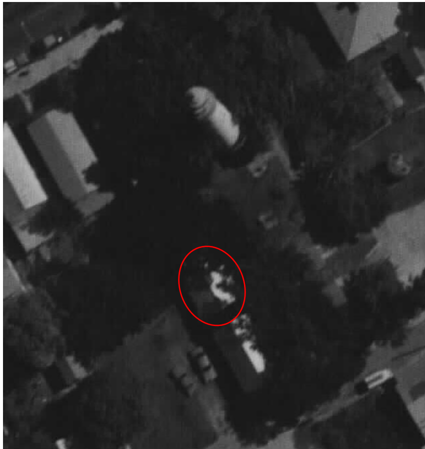
1972 Aerial Photo showing rear addition.
