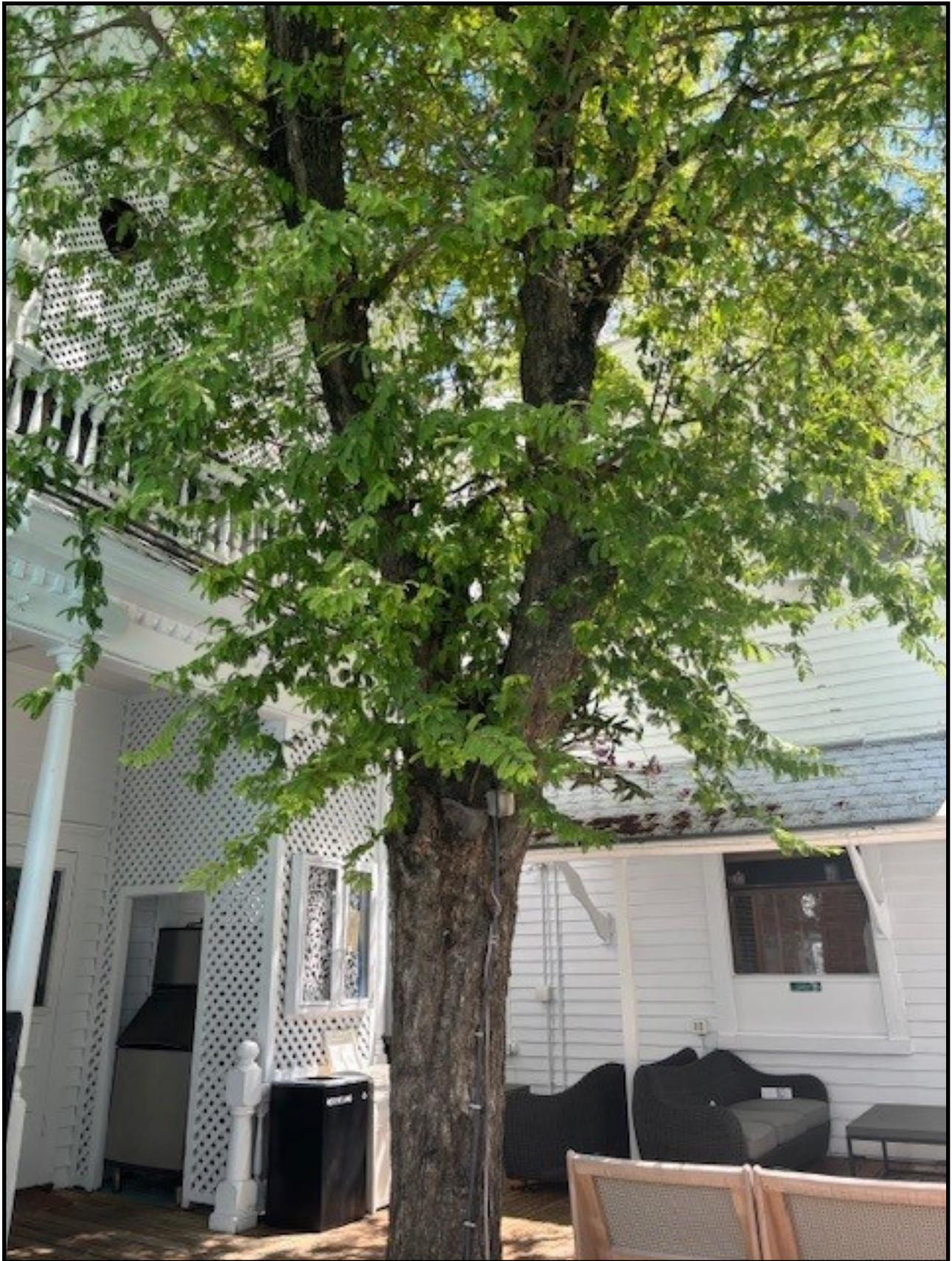
The canopy is very thin and included bark is present between the two competing leaders.
