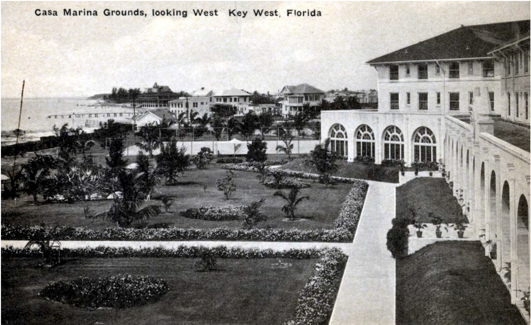
Casa Marina Hotel looking west from rear of building. No date available. The DeWolfe and Wood Collection. Monroe County Library.
