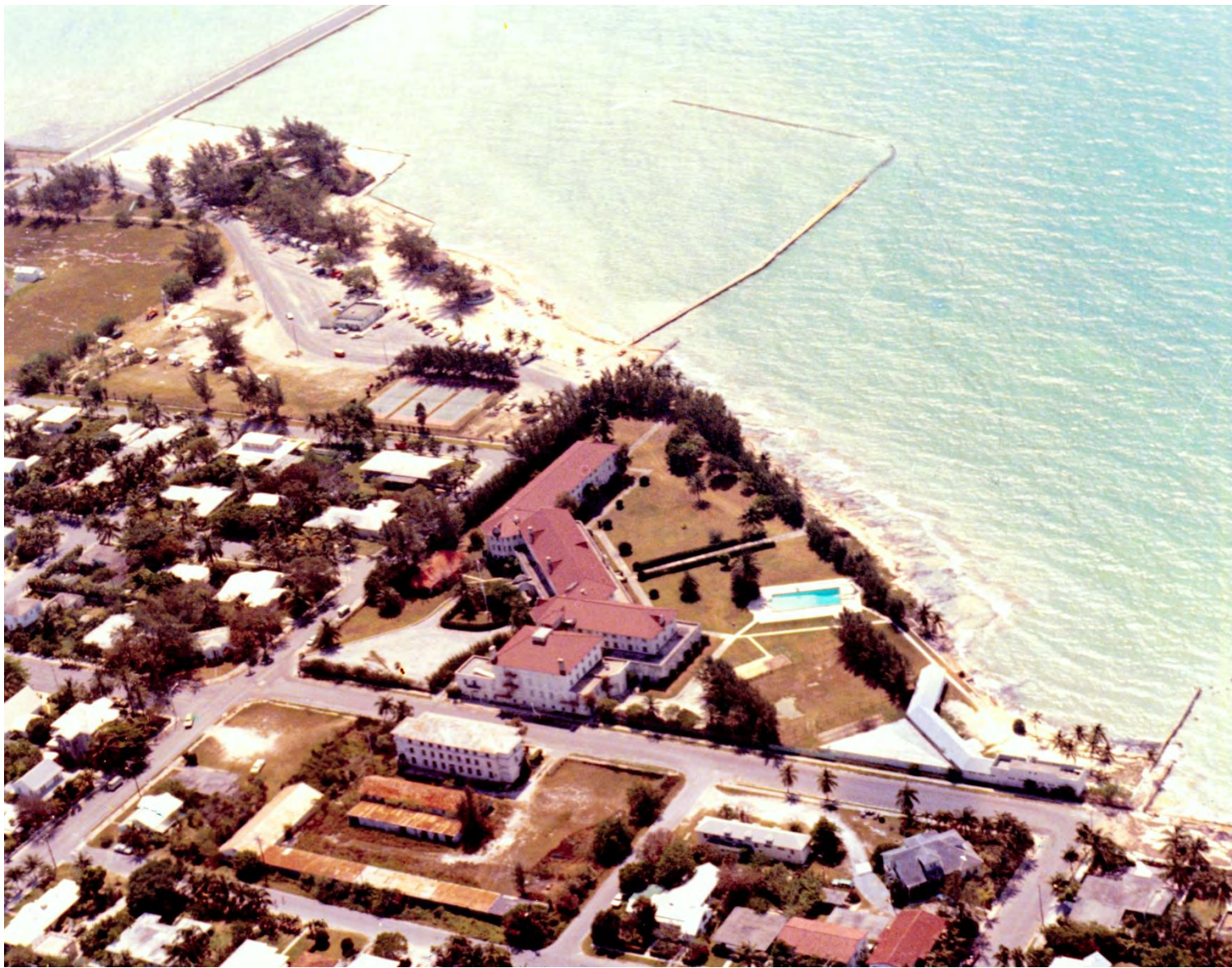
Aerial photograph of Casa Marina 1976. Monroe County Library.
