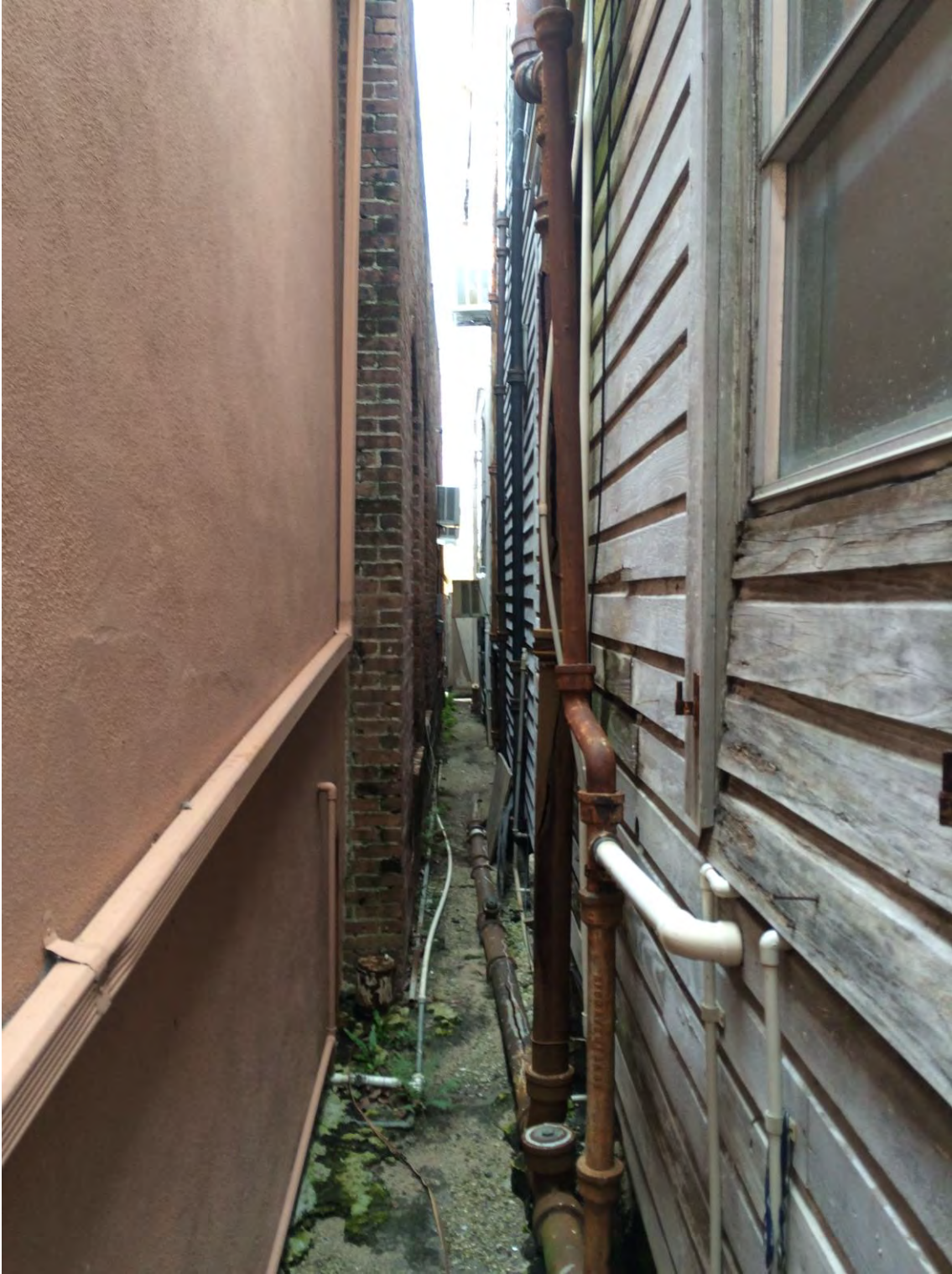
REAR OF 601 FLEMING AND SIDE OF 423 SIMONTON
