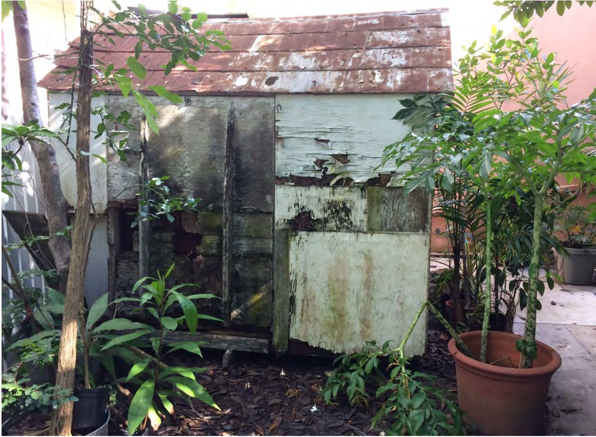
SHED TO BE REMOVED
