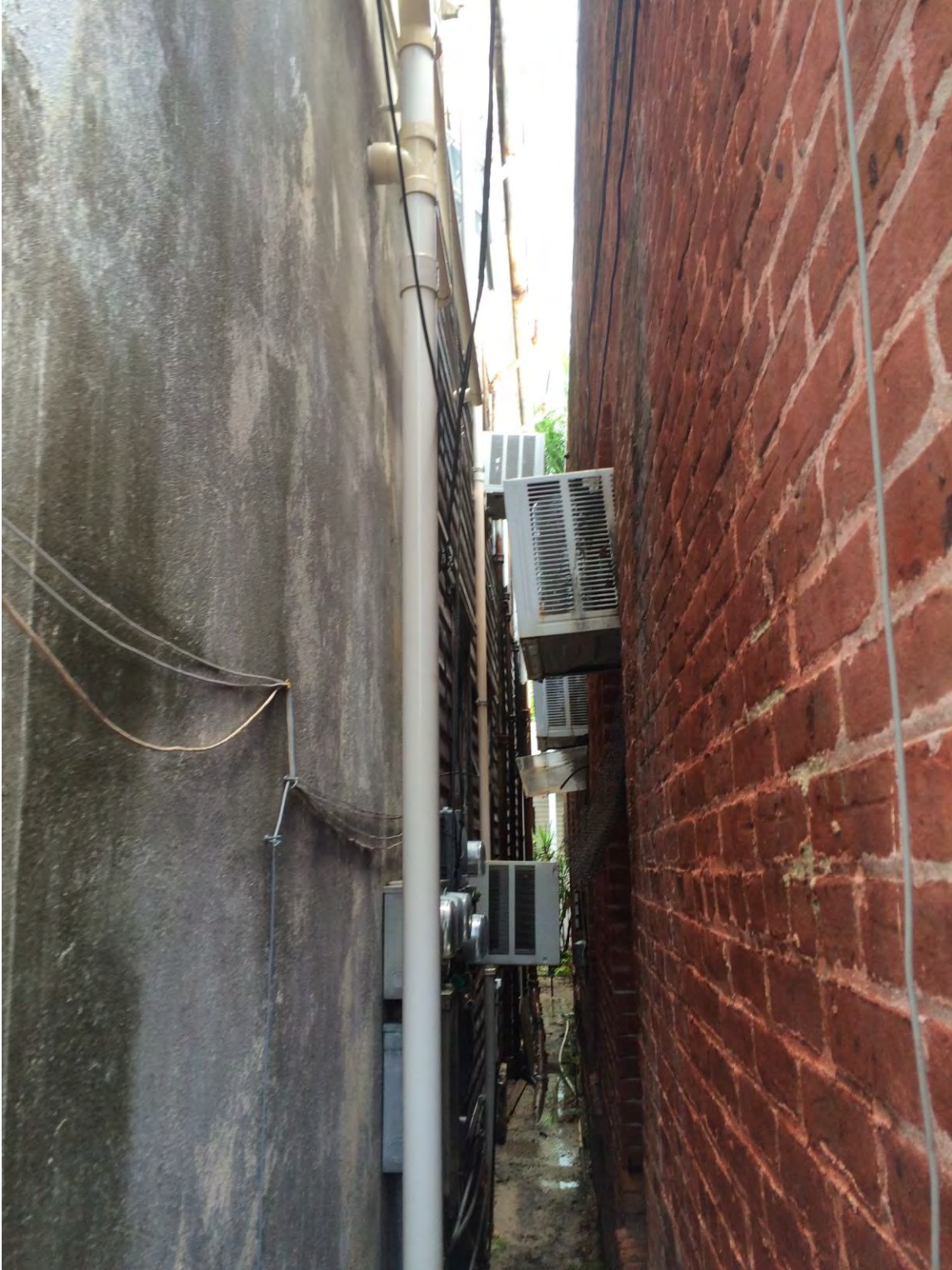
SIDE OF 423 SIMONTON AND REAR OF 601 FLEMING
