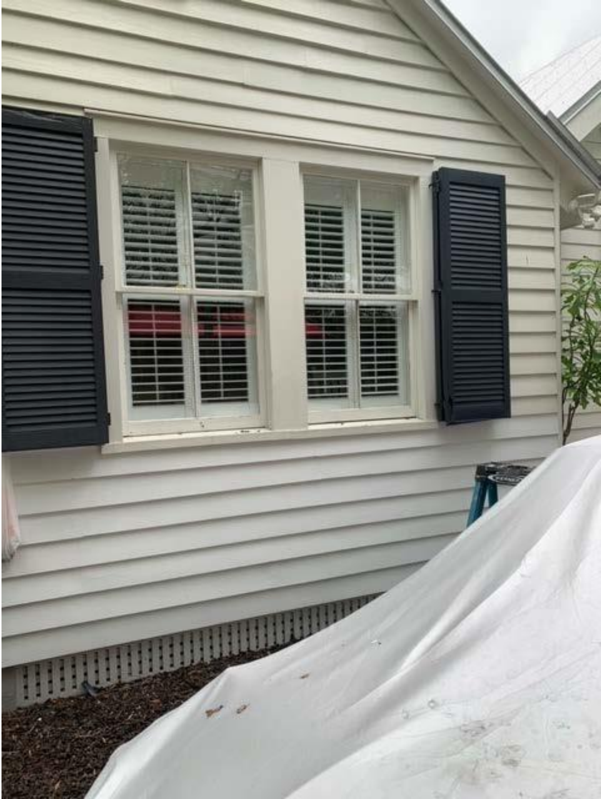
View 2 of windows on West elevation of 1012 Southard Street.
