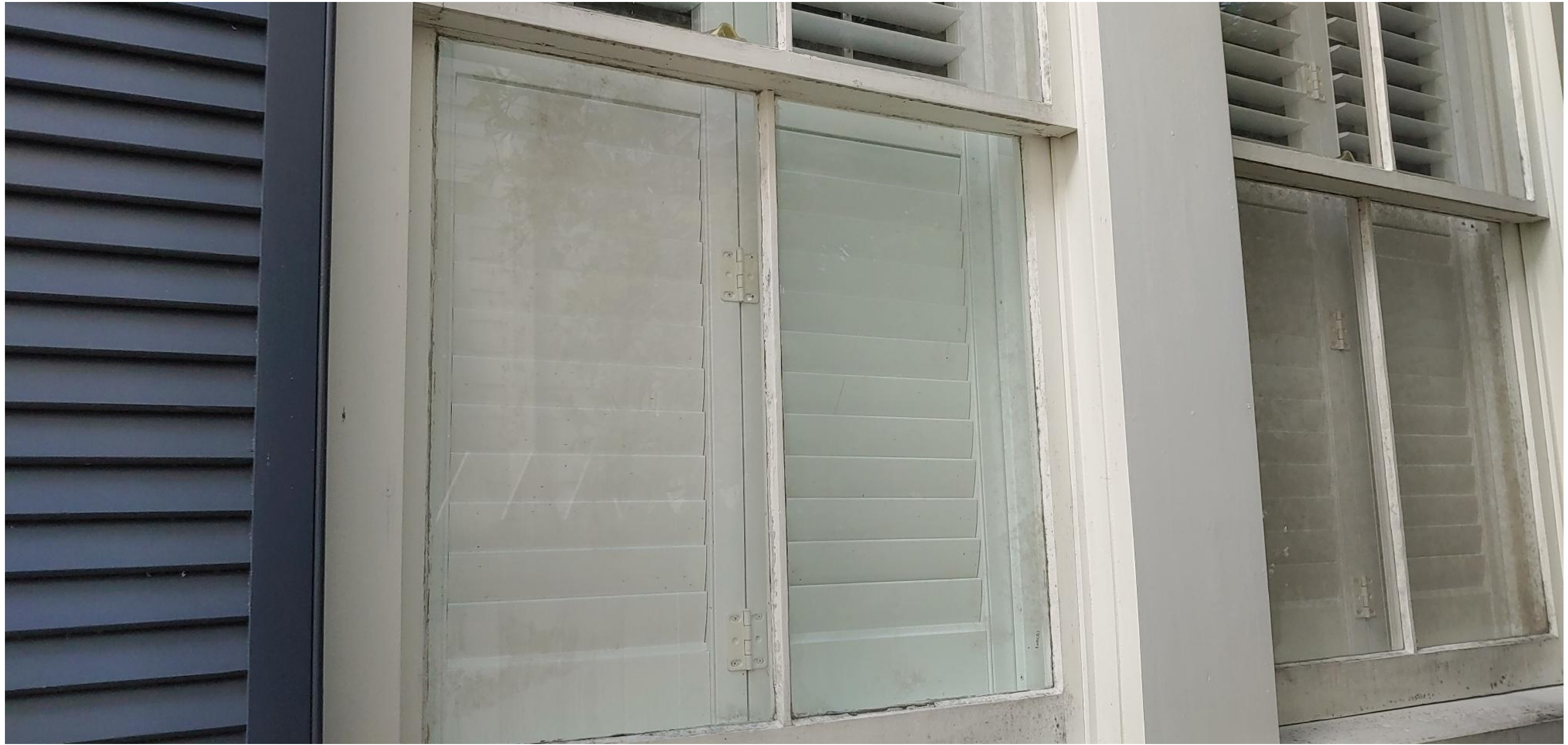
Windows on East Elevation 2. 1012 Southard Street. Photo by Brandon Celli.
