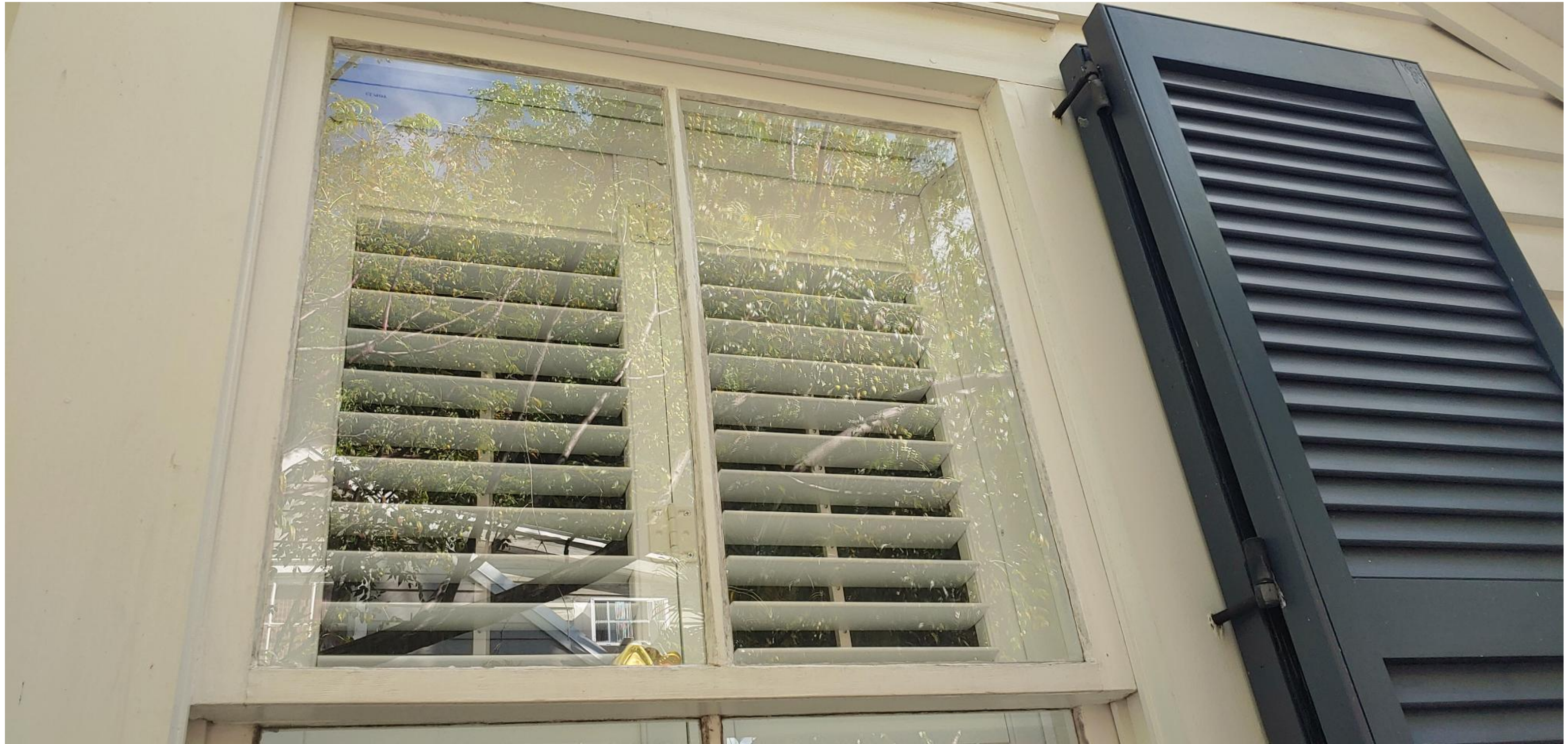
Up-close Window on West Elevation. 1012 Southard Street. Photo by Brandon Celli.
