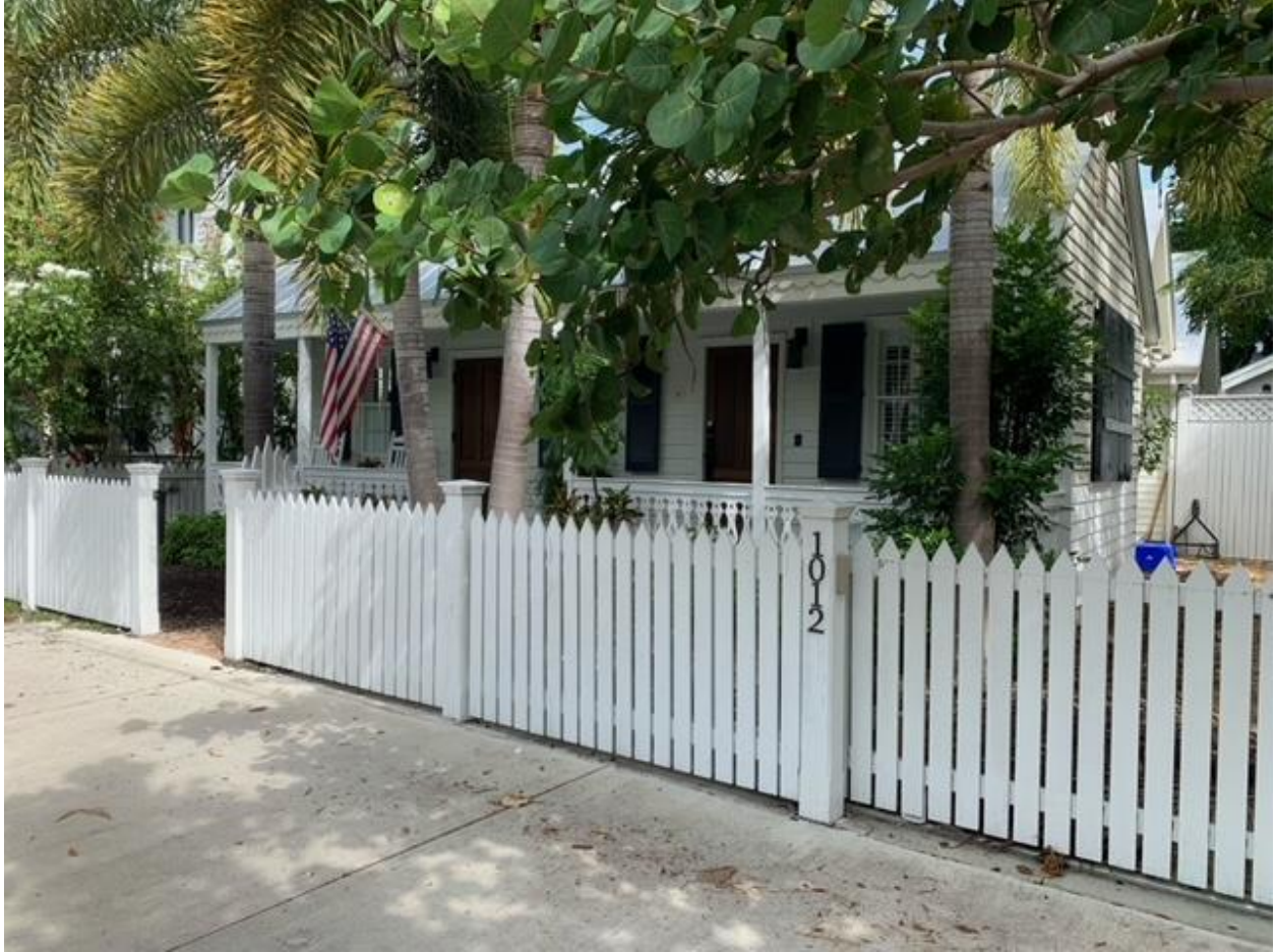
Front elevation view of 1012 Southard Street.
