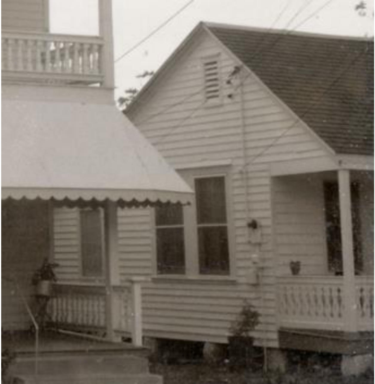
1965 photo showing the house at 1012 Southard Street. 2-over-2 windows visible on the side of the house and a 6-over-6 window visible on the front of the house.
