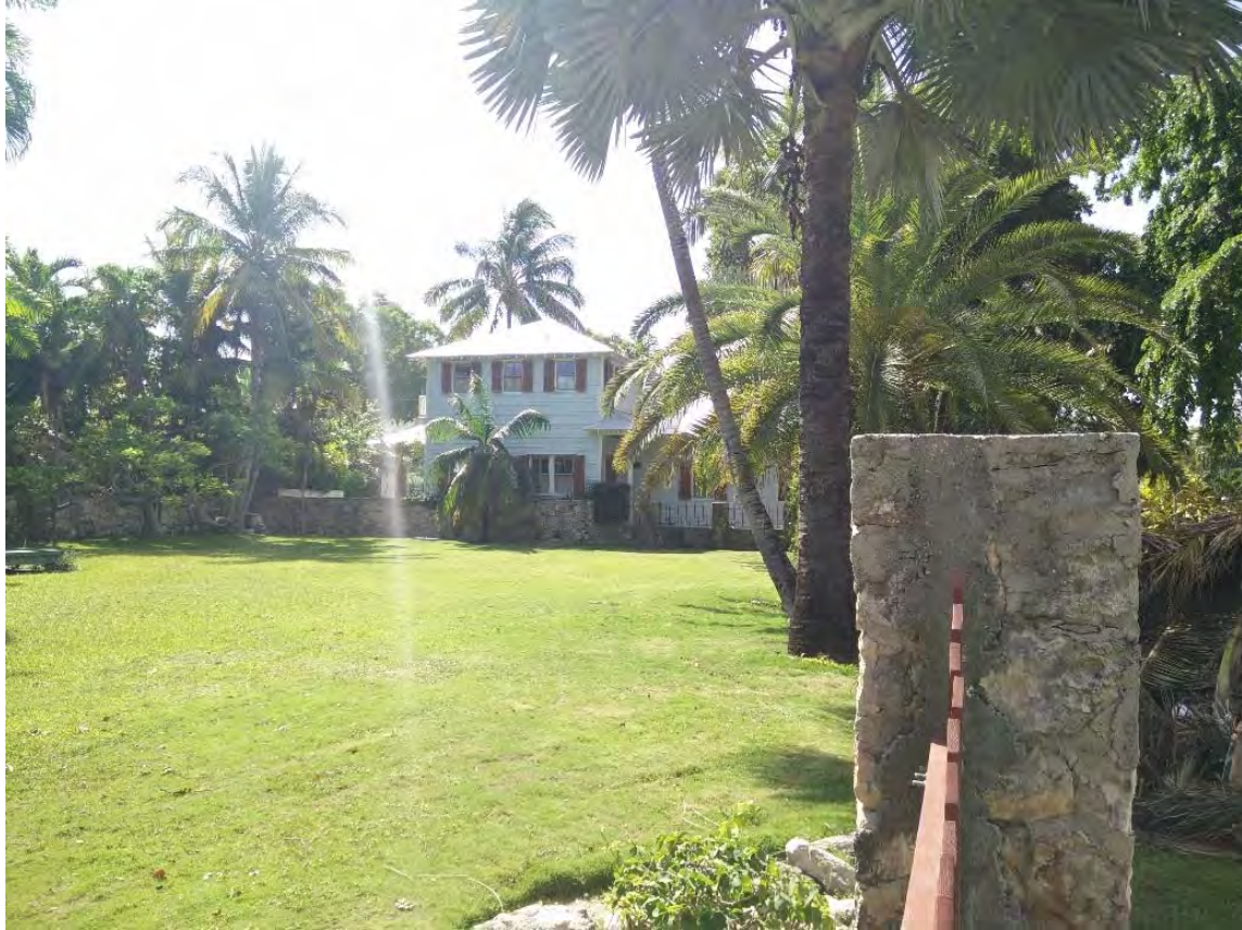
View of 1402 Whalton Street and adjacent house from Whalton Street
