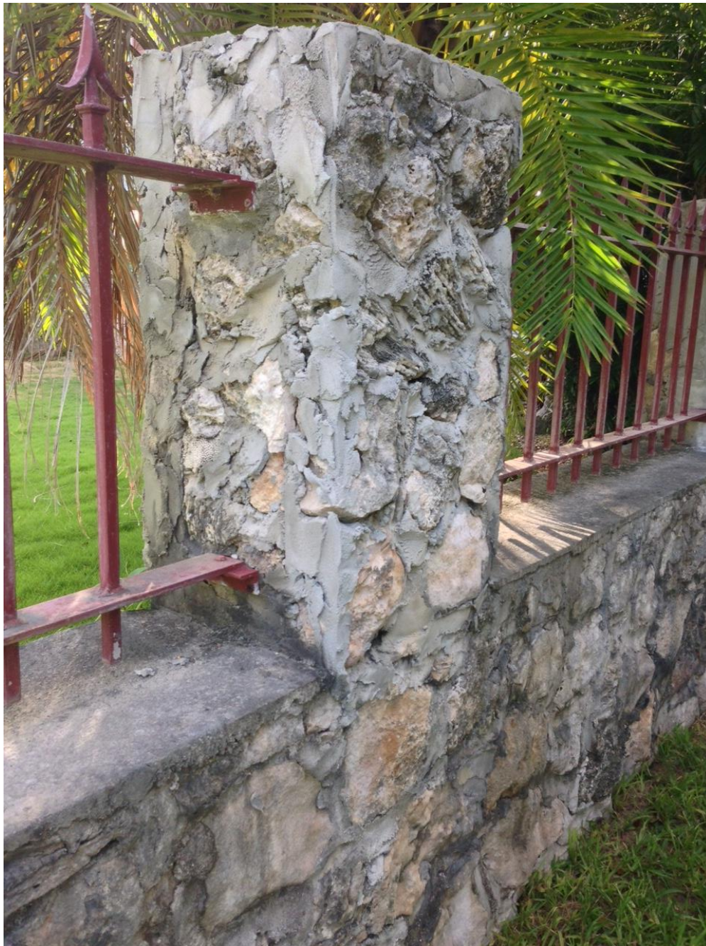
Portion of wall to be demolished.
