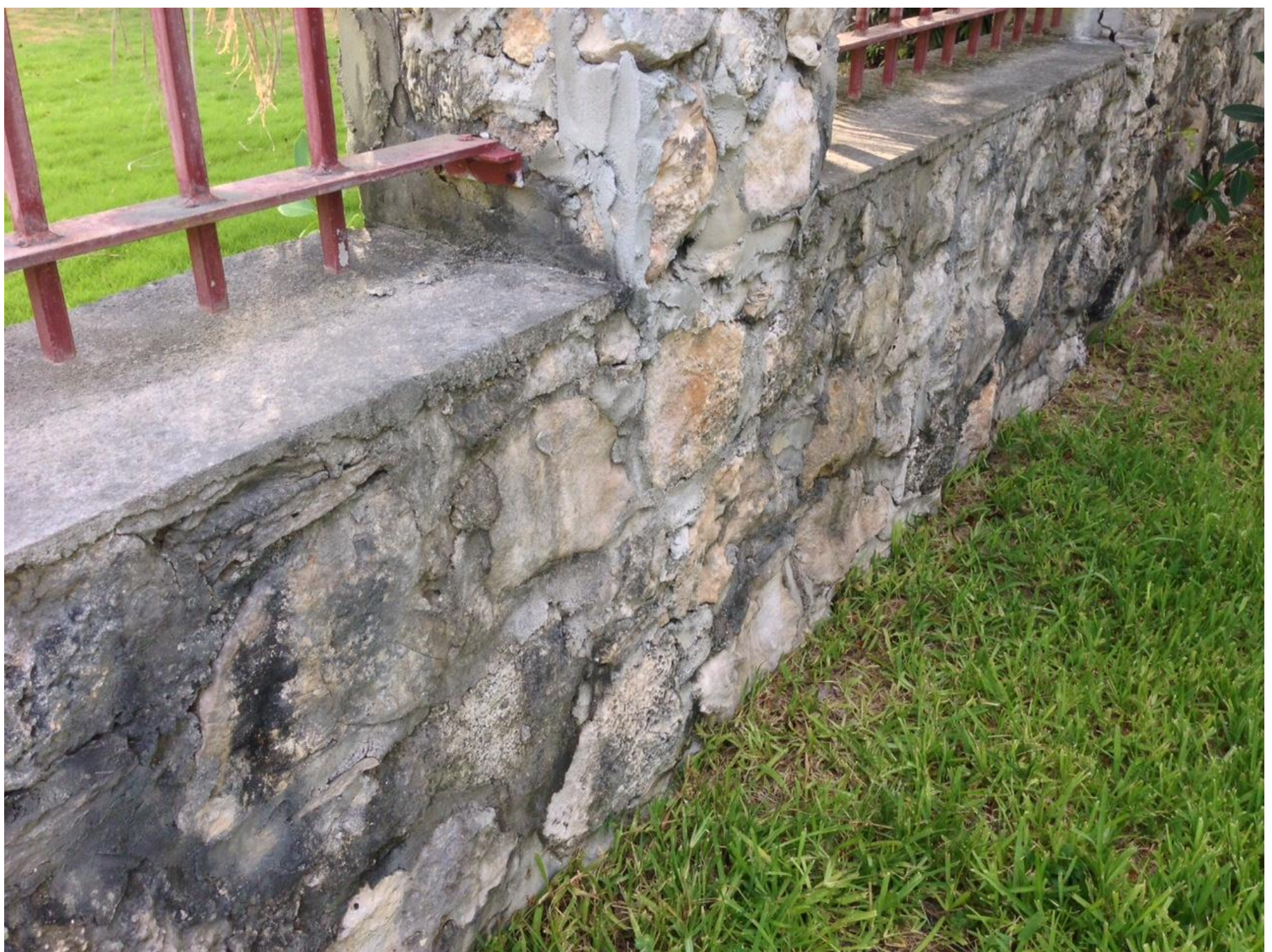
Portion of wall to be demolished.
