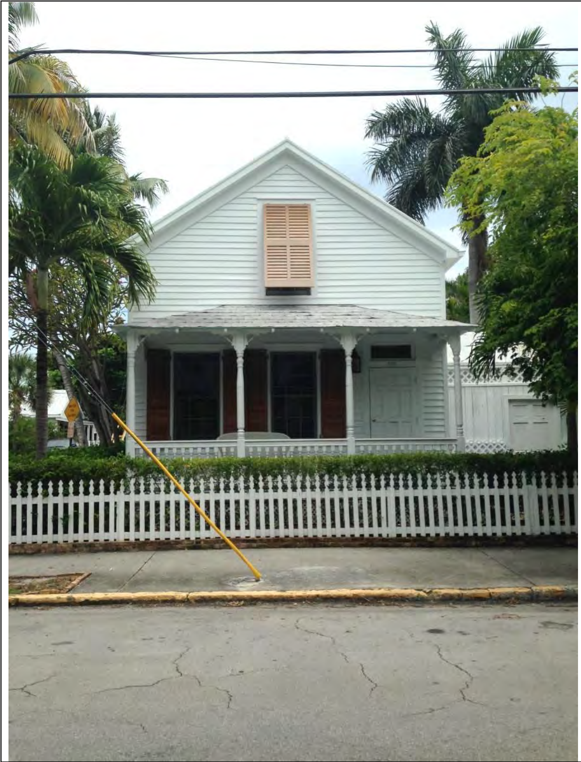
1. 1112 Southard Street. View from the street.
