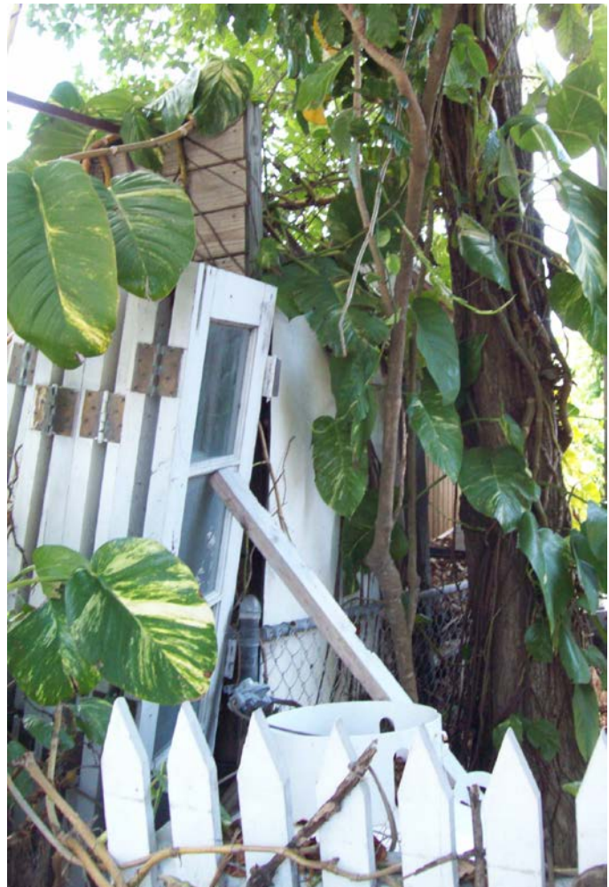
Fence falling into neighbor's yard
