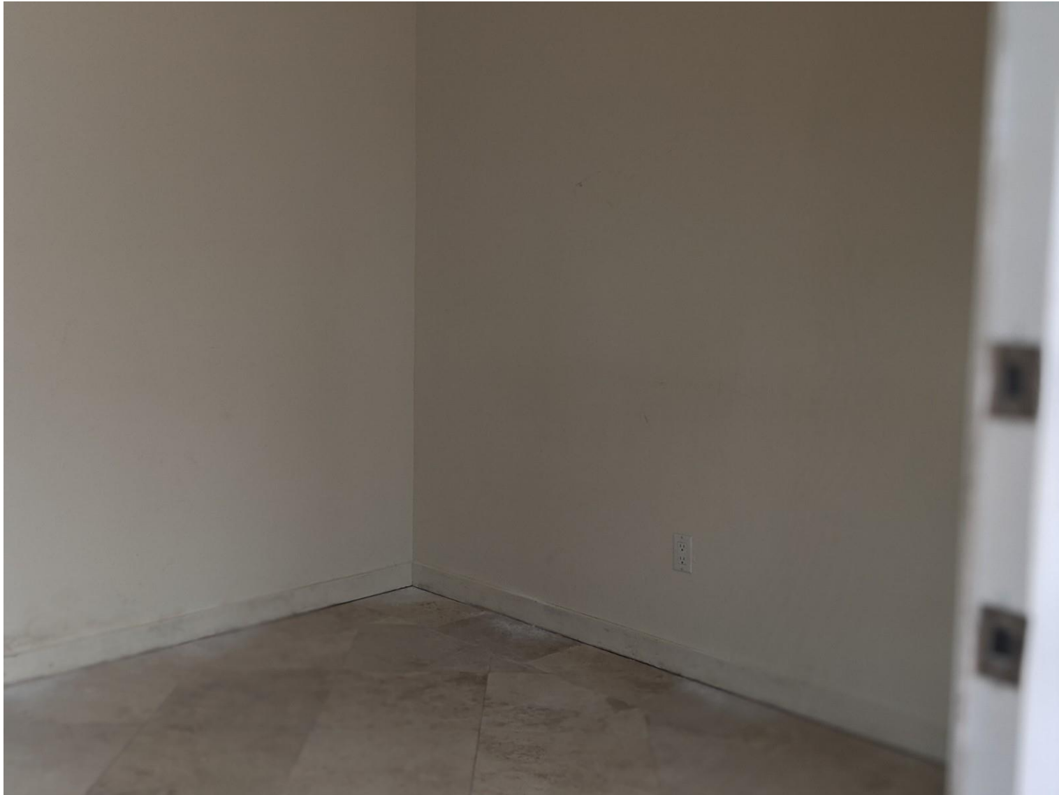
Interior space when entering the accessory structure.
