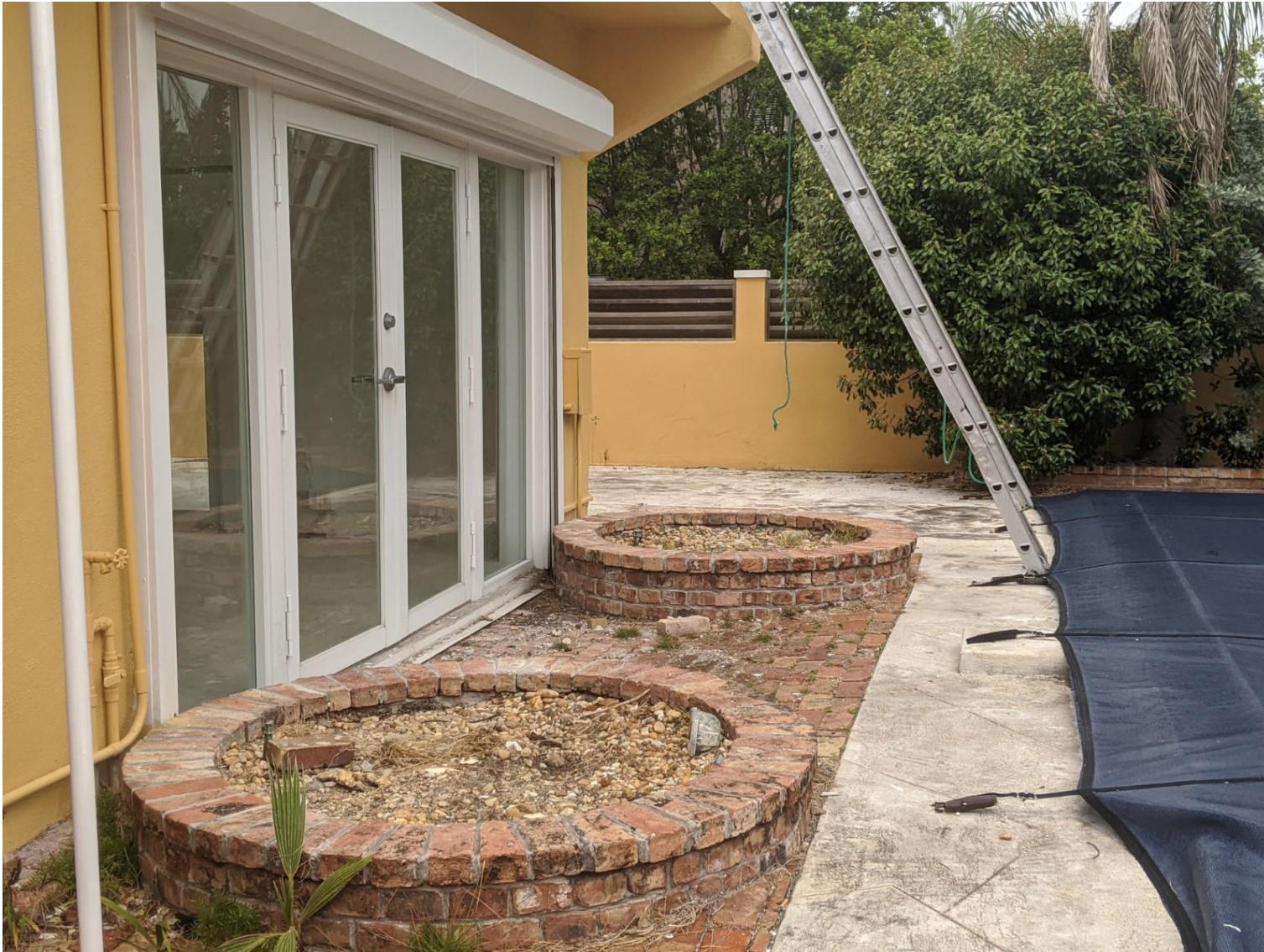
The entrance door to accessory structure facing the covered pool.
