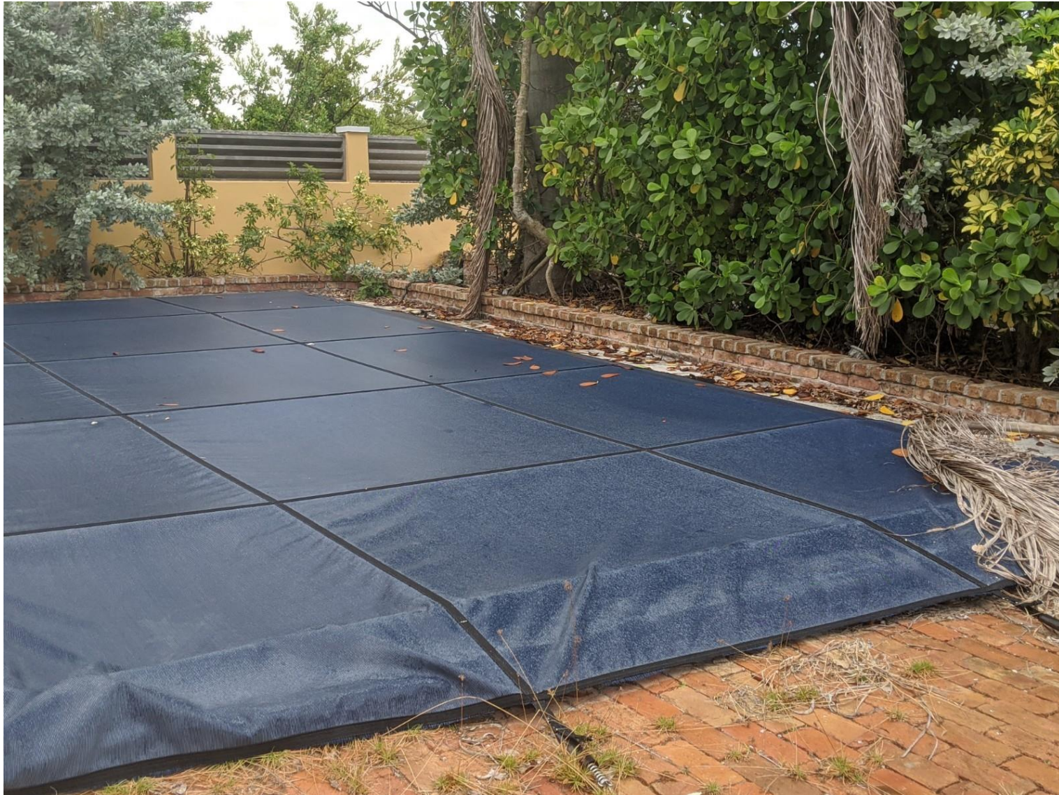
The existing covered pool facing the front entrance of the accessory structure.
