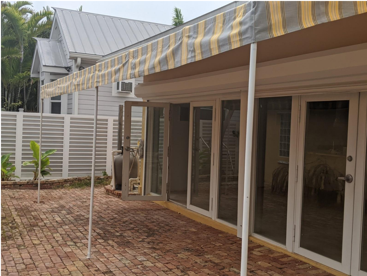
The rear exit/entrance to the principle structure.
