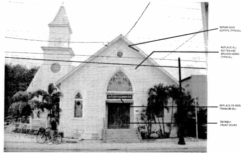
TRUMAN AVENUE VIEW (FRONT OF CHURCH)
