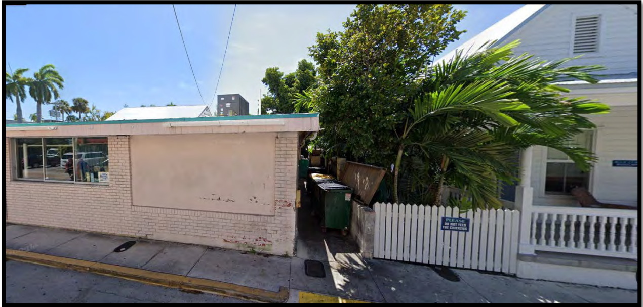
Streetside (Catherine) & Rear (Southwest) Elevation
