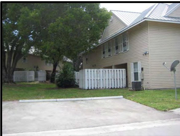
VIEW OF REAR ELEVATION OF TYPICAL SUBJECT BUILDING
