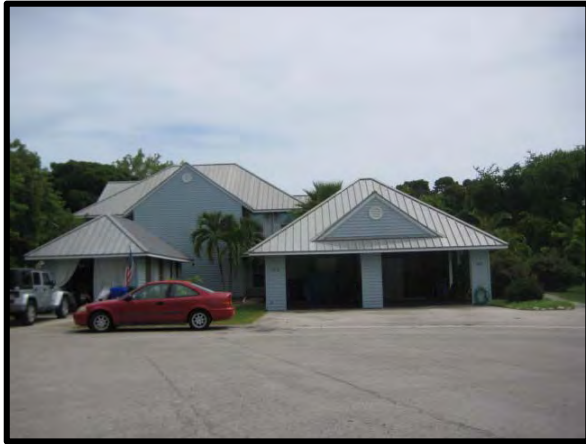
VIEW OF TYPICAL SUBJECT BUILDING
