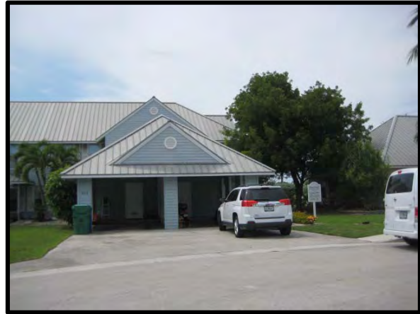
VIEW OF TYPICAL SUBJECT BUILDING
