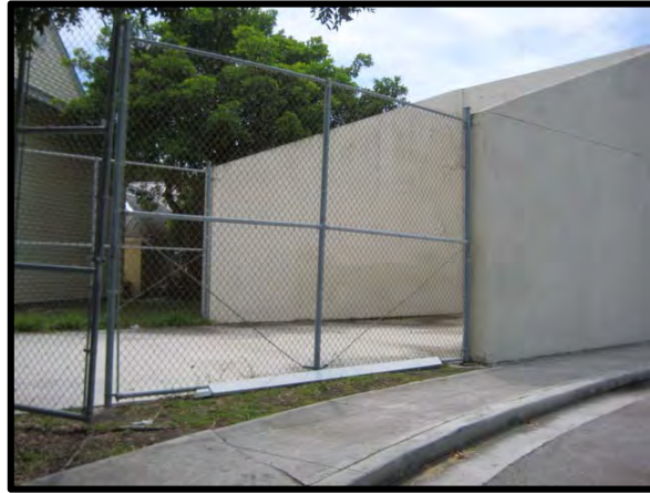
VIEW OF SUBJECT PROPERTY RACQUETBALL COURT
