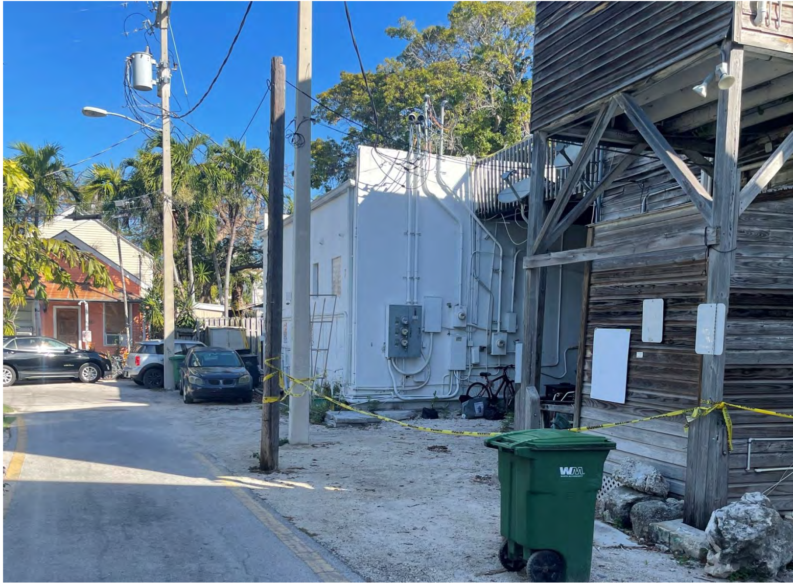
7 ARONOVITZ LANE LEFT NEIGHBORING PROPERTY SIDE VIEW
