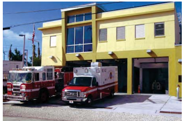
Conch Key Fire Station, Conch Key, FL
