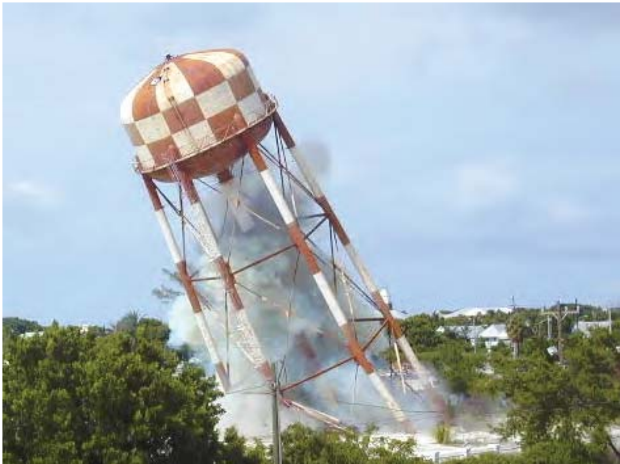
Water Tank Demolition, NAS Key West
