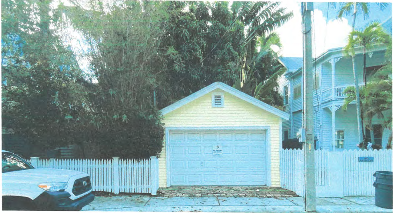
620 Dey Street - Garage
