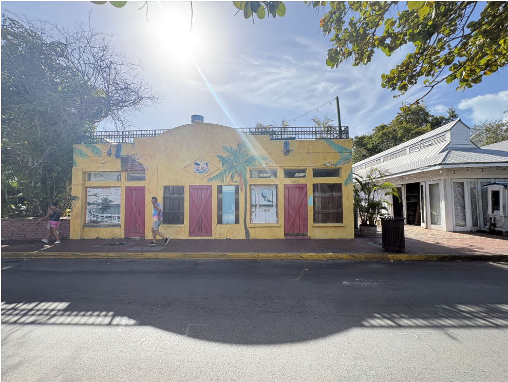
324 PETRONIA ST. | North elevation #2 [2026.03.10].
