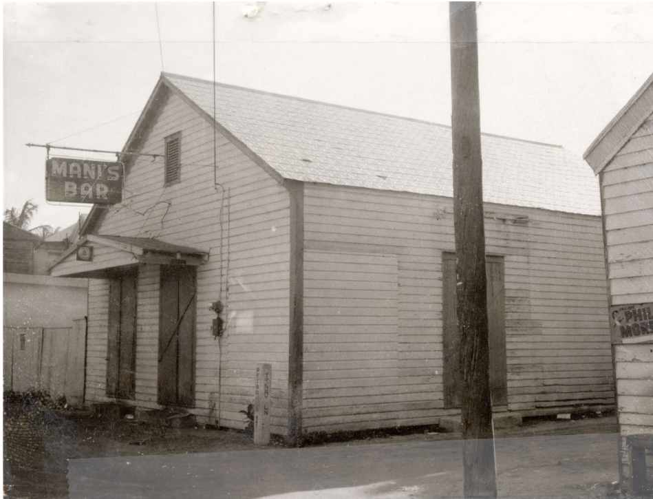
316 PETRONIA ST. | 1965 Monroe County Property Appraiser. Note: differences in siding demonstrate where former fenestrations / openings once existed.
