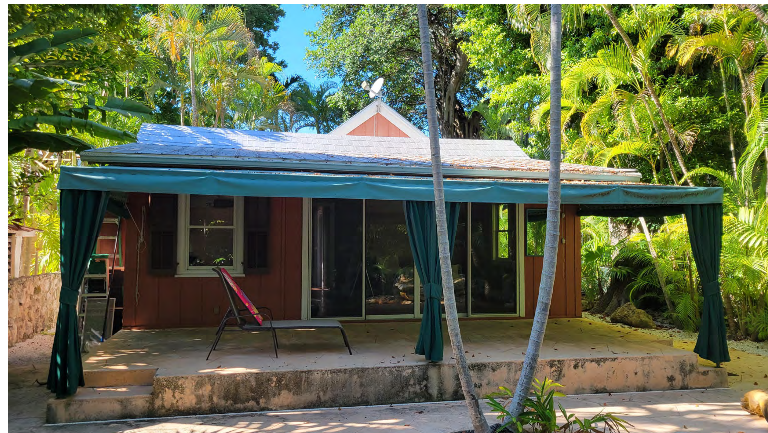
REAR ELEVATION FACING SOUTH
