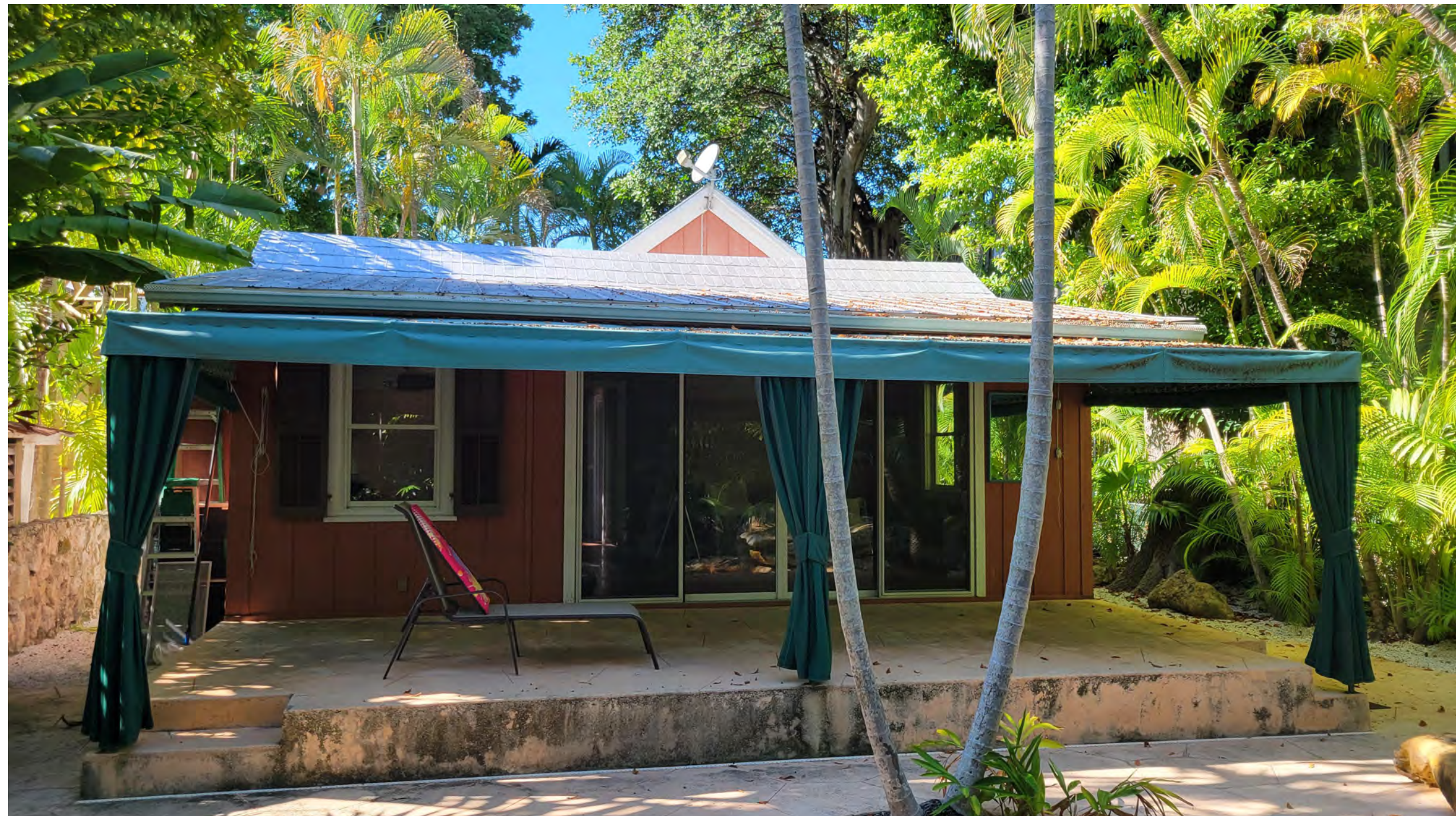
REAR ELEVATION FACING SOUTH
