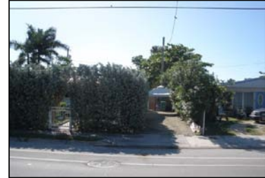
Sample of view of tap pole
