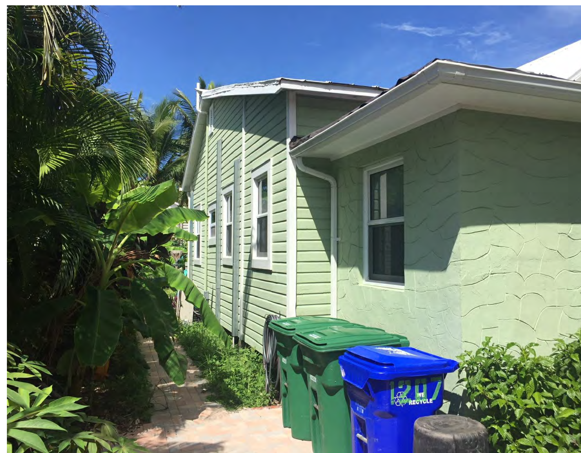
2 PHOTO OF SOUTH FACADE (SIDE YARD)
