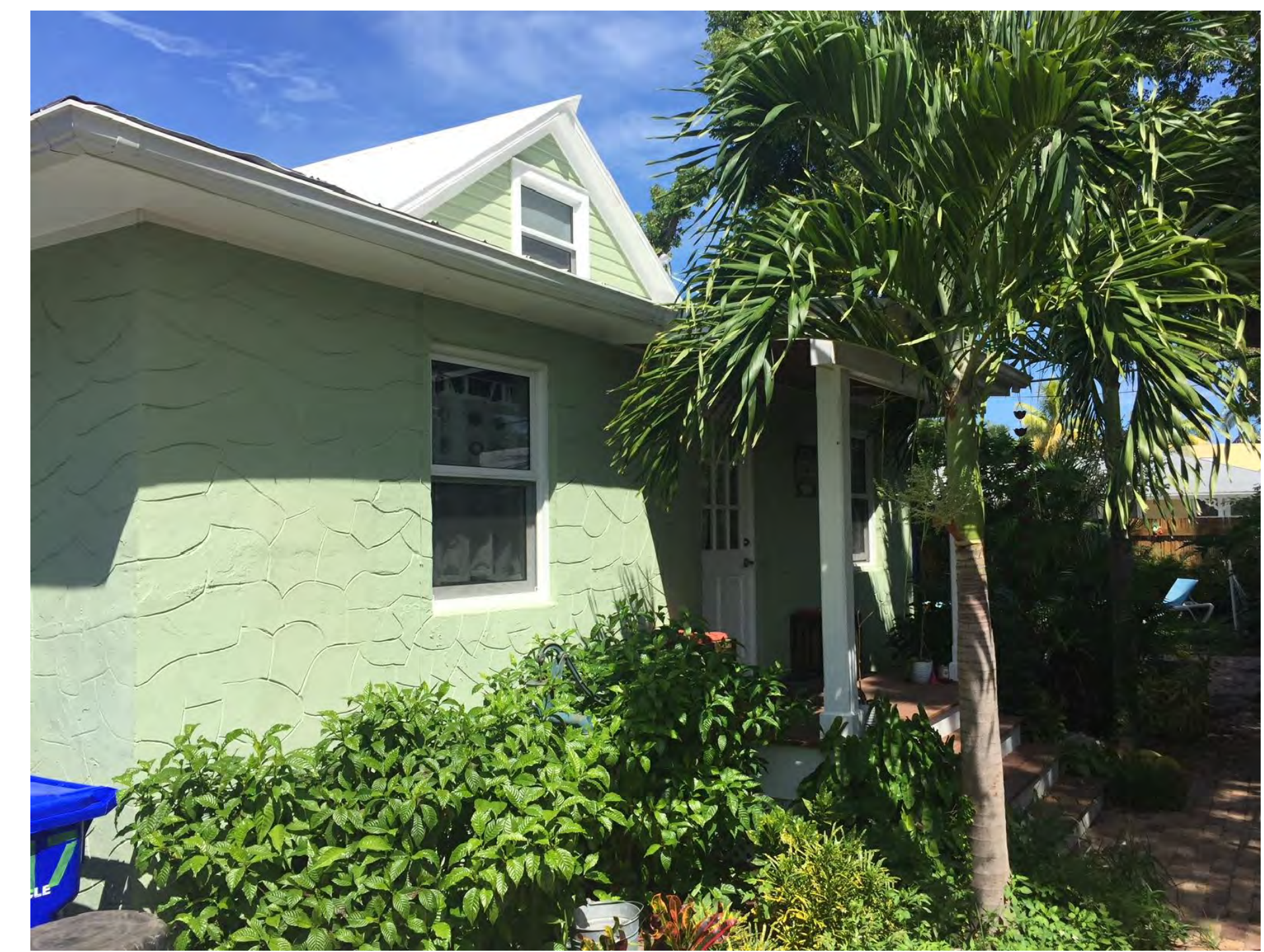
1 PHOTO OF GEORGIA STREET FACADE (EAST FACADE)
