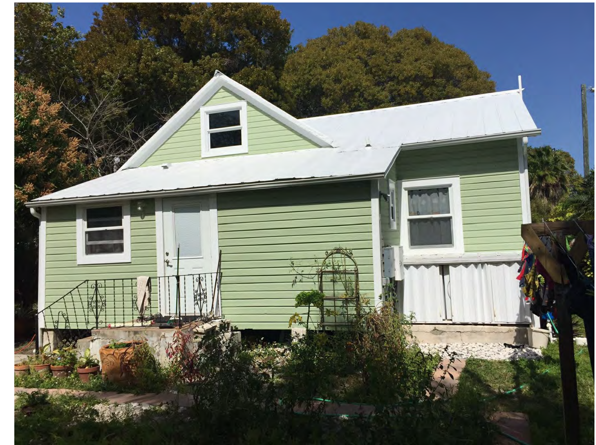
4 PHOTO OF WEST FACADE (REAR YARD)
