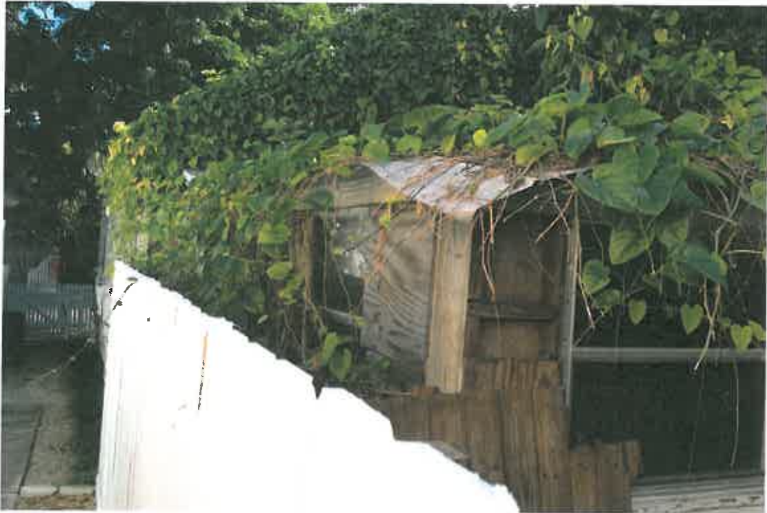
NORTHWEST SIDE LOOKING FROM REAR
