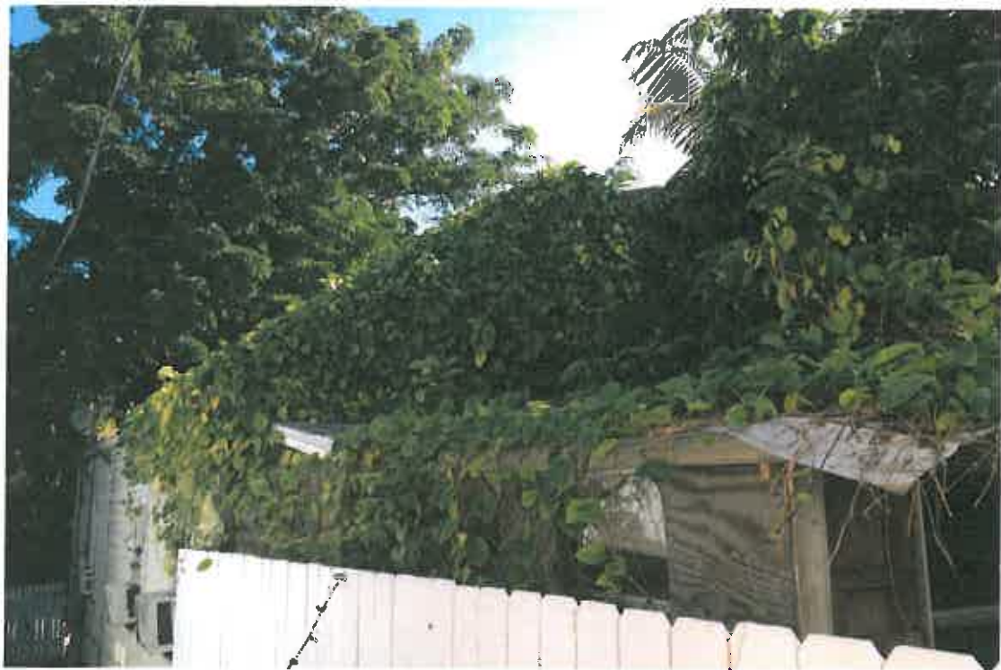
NORTHWEST SIDE LOOKING FROM REAR
