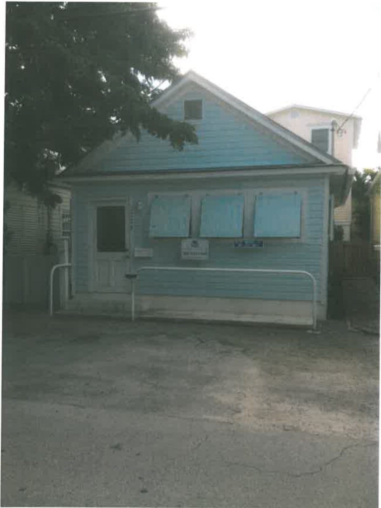
NEIGHBORING HOUSE TO THE WEST - 1220 GRINNELL
