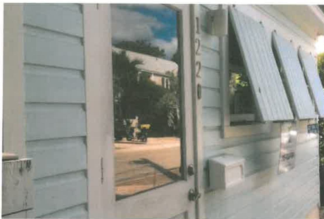
NEIGHBORING HOUSE TO THE WEST - 1220 GRINNELL
