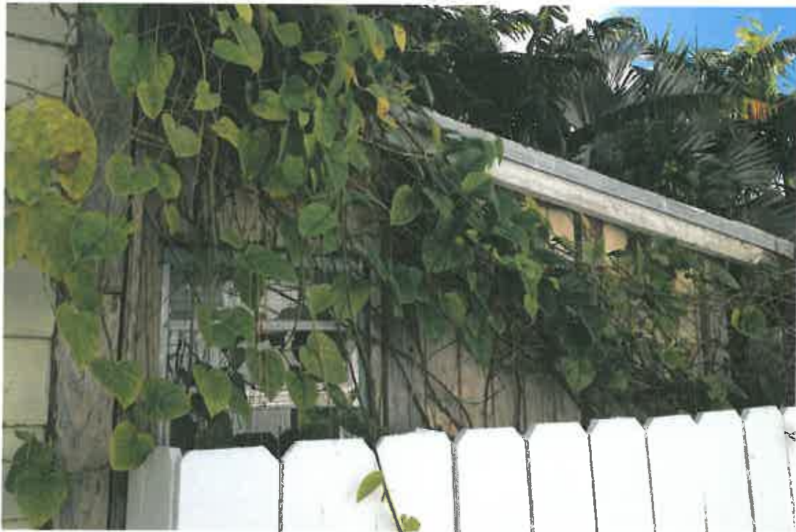
NORTHWEST SIDE OF REAR ADDITION
