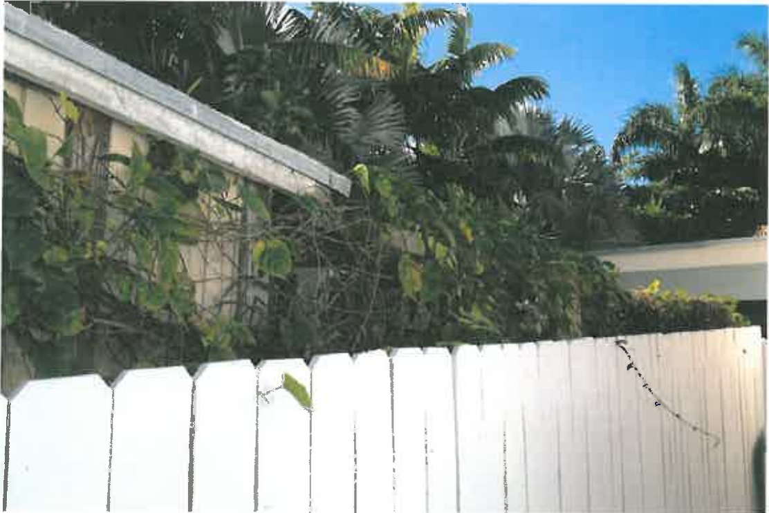
NORTHWEST SIDE OF REAR ADDITION
