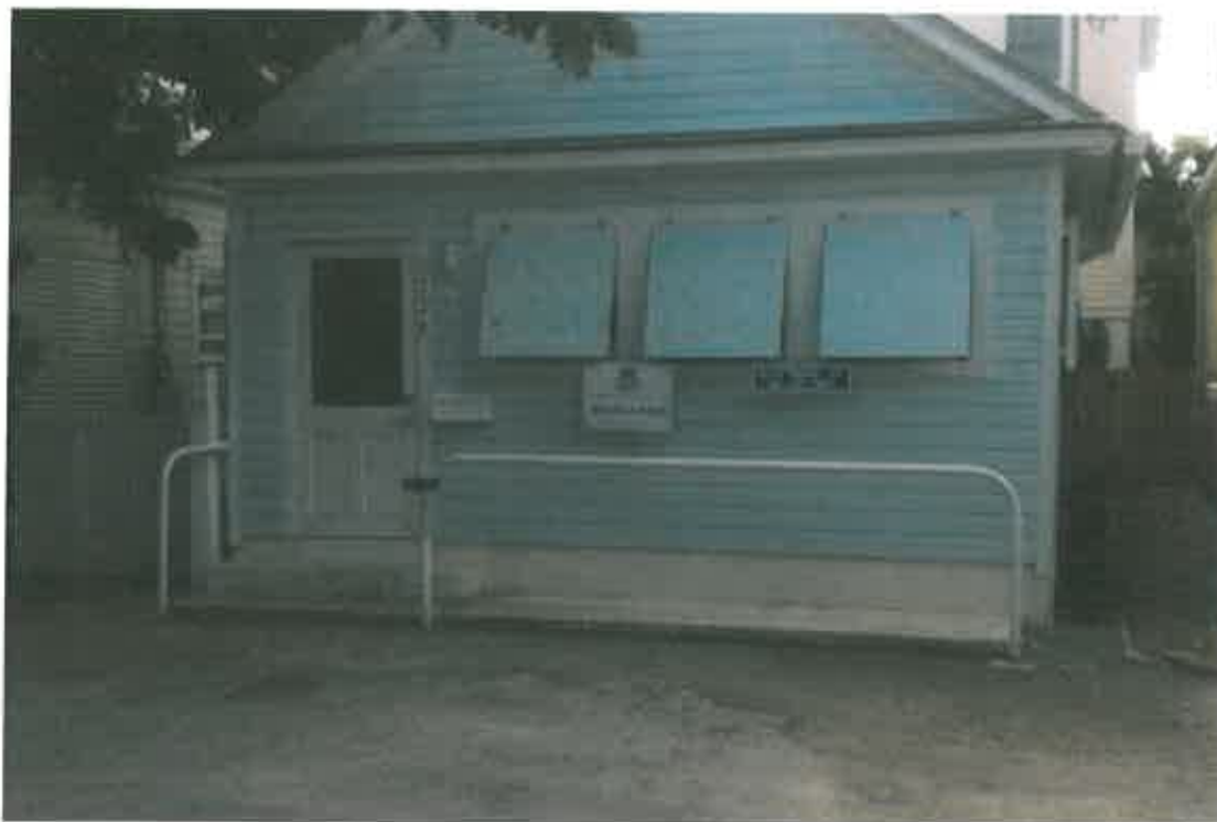
NEIGHBORING HOUSE TO THE WEST - 1220 GRINNELL
