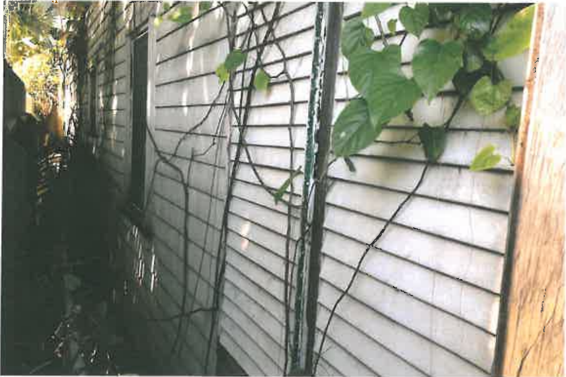
SOUTHEAST SIDE LOOKING FROM FRONT
