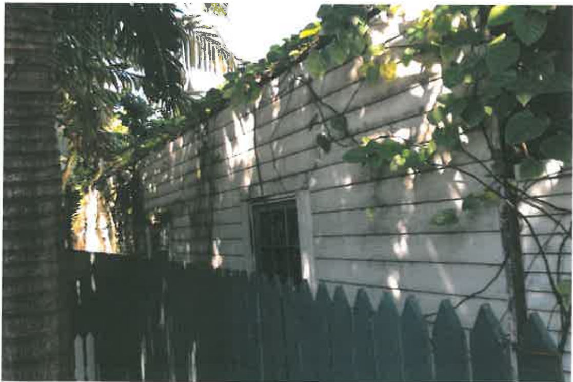
SOUTHEAST SIDE LOOKING FROM FRONT
