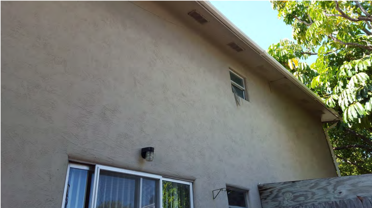
Back of Rear Building
