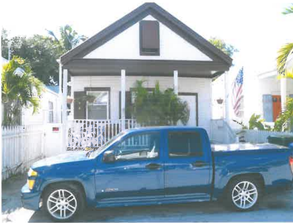
712 Chapman Lane - Adjacent Property
