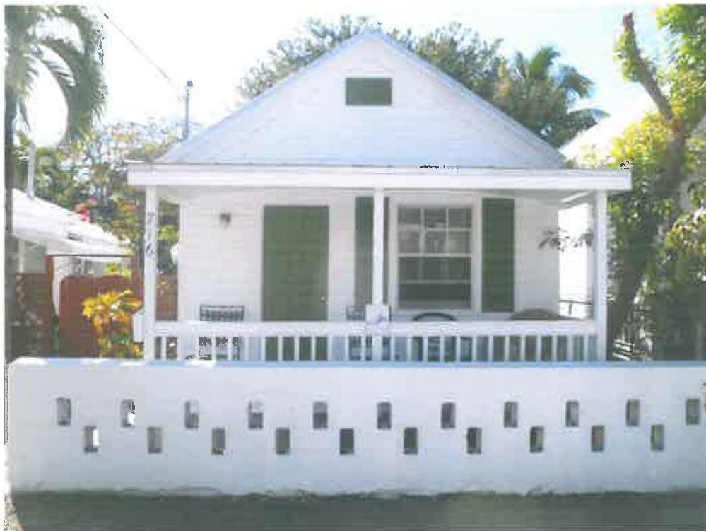
716 Chapman Lane - Adjacent Property
