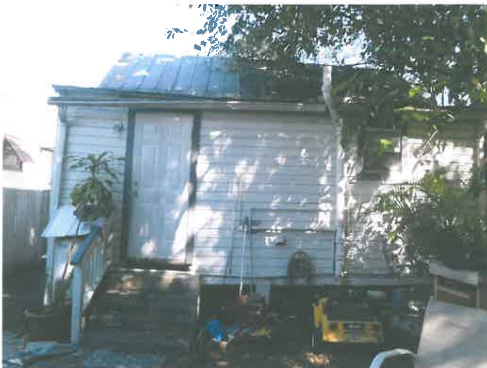
714 Chapman Lane - Rear structure to be removed
