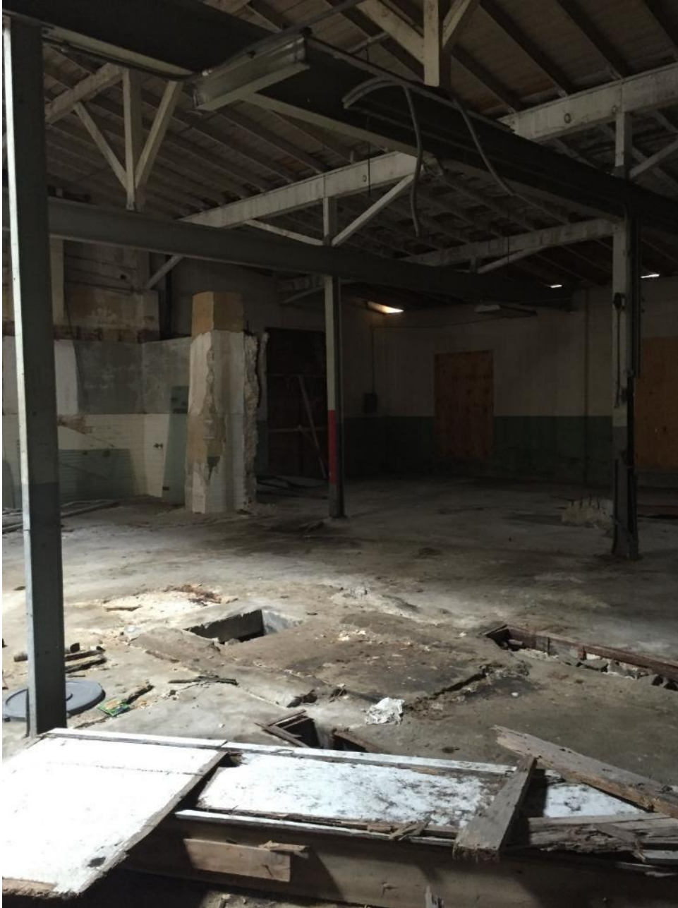
PHOTO 1: Interior of buildings at the Site
