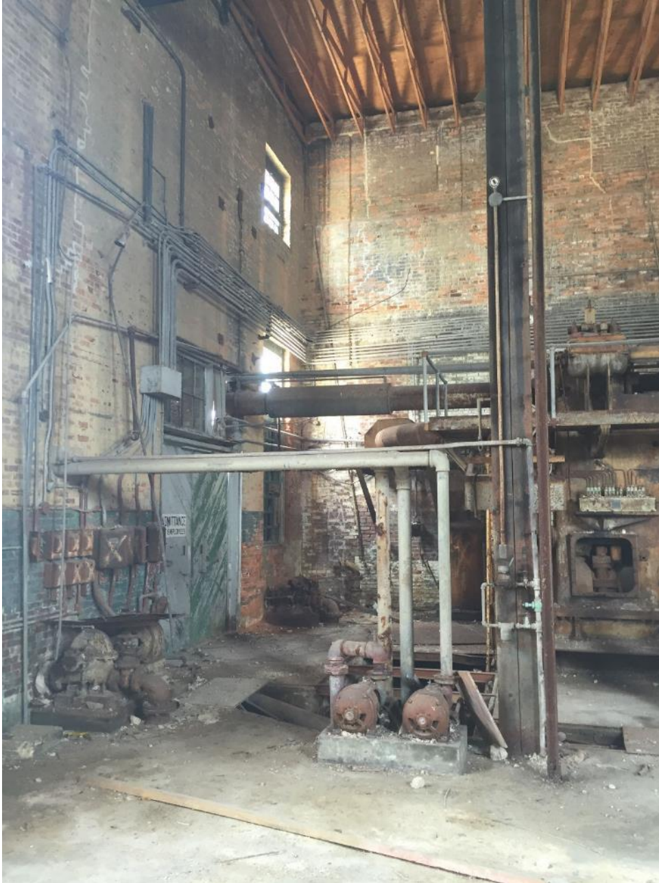
PHOTO 7: Interior of buildings at the Site
