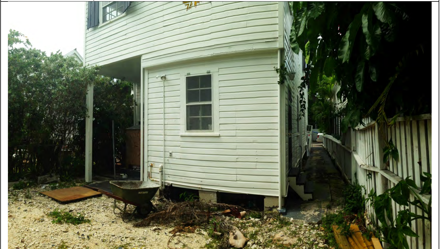
4. 808 Olivia Street- Rear Elevation View
